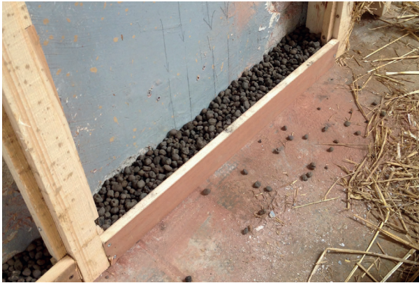
Figure 60. Expanded clay used to fill the space between floor and the light earth insulation. Photo: Arthur Bohn
