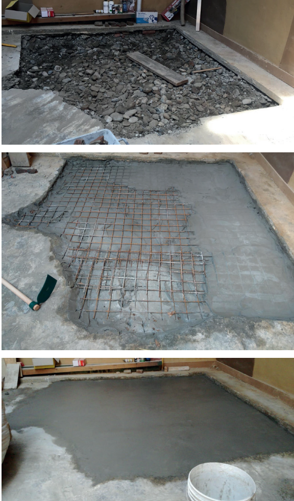
Figure 39, 40 and 41. One of the voids in the Red Room's floor getting filled with a reinforced concrete mix.
