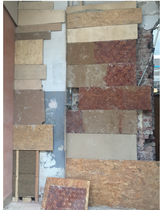
Figure 154. The different boards used for the shutterings on the right side of the wall.
