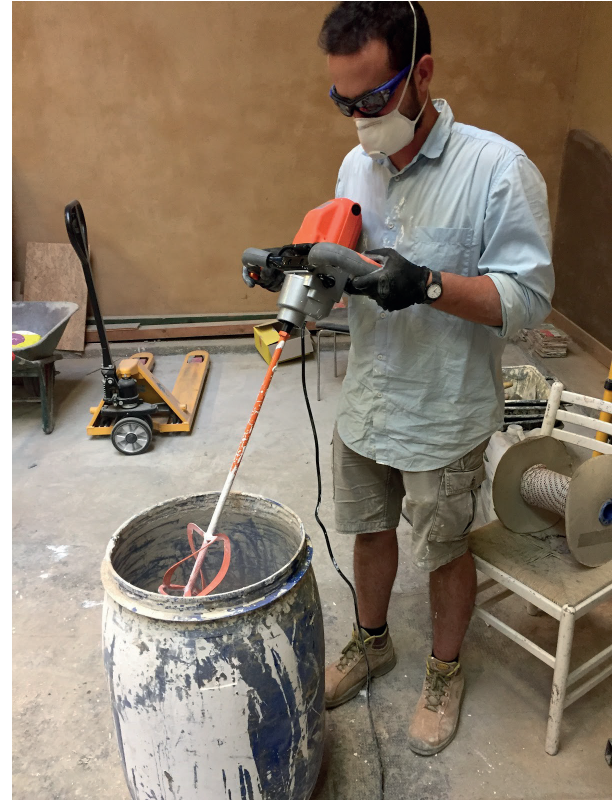
Figure 151. Waterproof gloves, protective goggles and a face mask are suggested to avoid possible skin irritations or problems the lime dust can cause to the eyes and the respiratory system. Photo: Andi Dani
