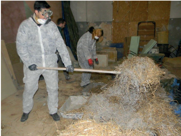
Figure 93. Students at work, mixing the dry straw with the soaked straw.
