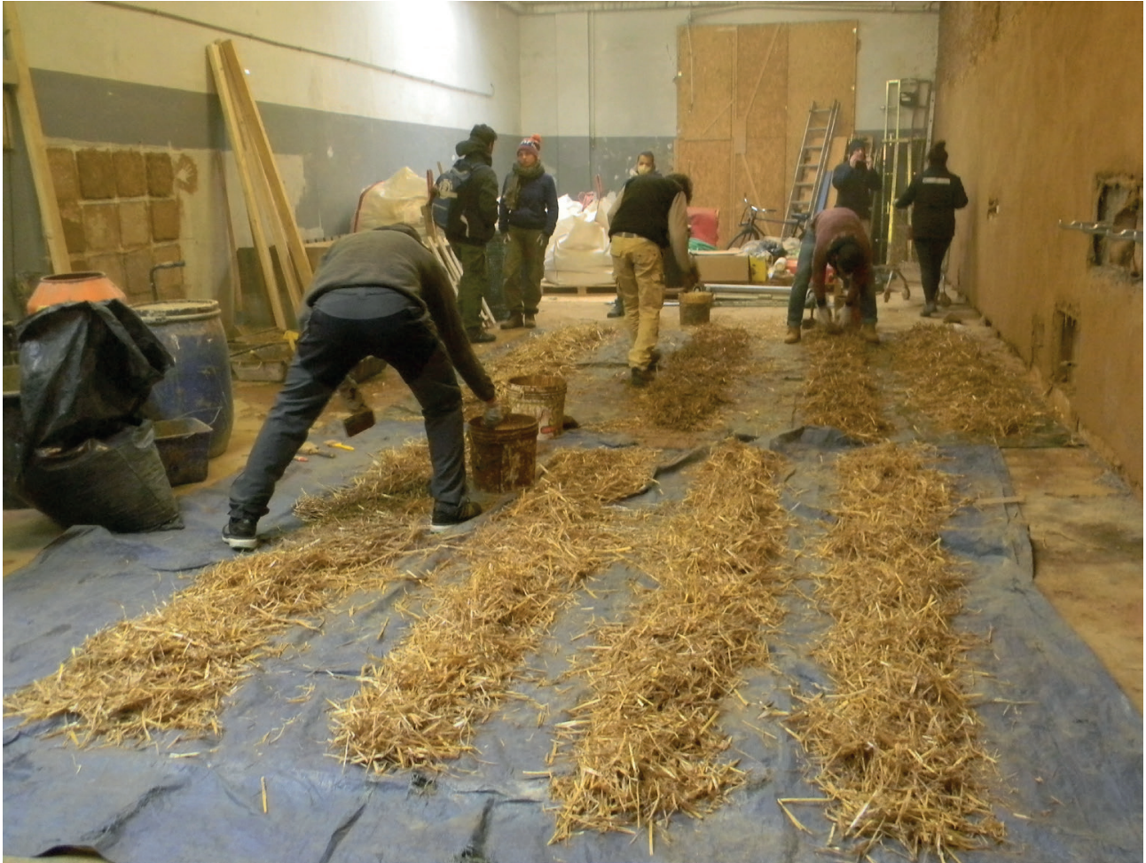
Figure 70. Straw was initially spread over impermeable bags and then clay slip was gradually poured over it. Photo: Jasenko Spahic
