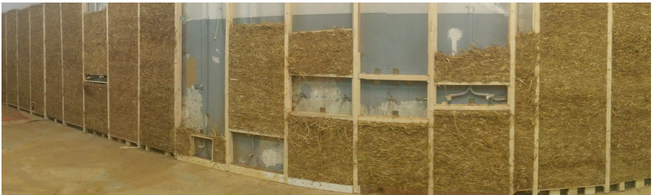
Figure 79. Straw and clay insulation as applied in the Red Room. View of the eastern wall. Photo: Nicoletta Palama
