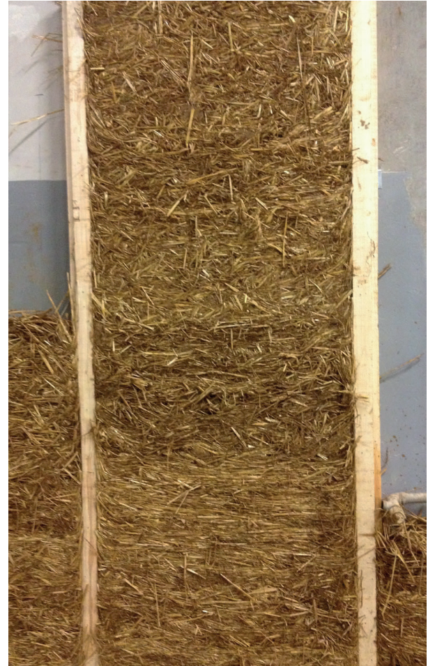
Figure 61. Light earth as applied in the Red Room. Photo: Nicoletta Palama
