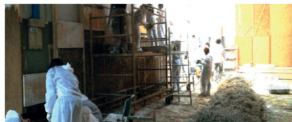
Figure 103. The casting process carried out by the students during the workshop of 23 May 2017. The lime straw mixture was initially laid over the wooden pallets for a short draining, and subsequently inserted in the shutterings.
