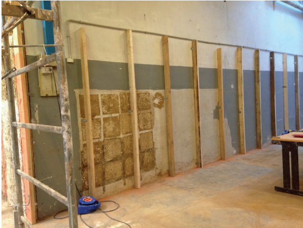
Figure 87. The lower part of the wooden skeleton with the vertical joists fixed on the eastern wall.
