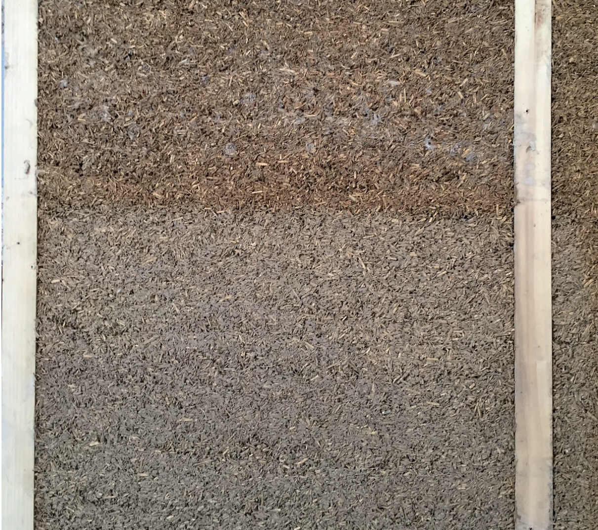
Figure 155. Keeping the shutterings for several days after the cast of hempcrete can result in mold manifestation (above) and a very slow drying process (below).
