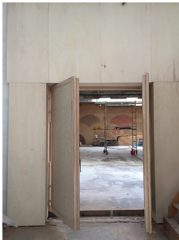
Figure 44. The south wall from the Officine Creative after the hemp door was built and fixed. Photo: Andi Dani
