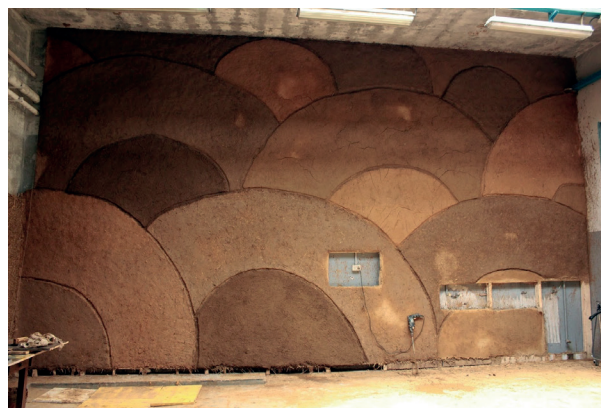
Figure 25. The north wall after the implementation of light earth and the raw earth plaster Photo: Arthur Bohn
