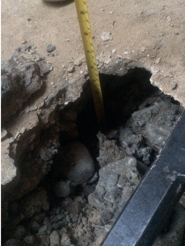
Figure 14. One of the spots where the floor was unstable and had cracked.
