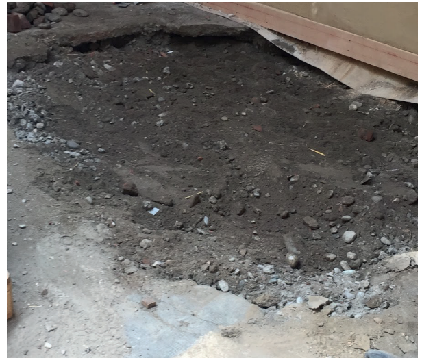
Figure 13. The void in the floor was covered with raw earth in order to level it. Photo: Andi Dani
