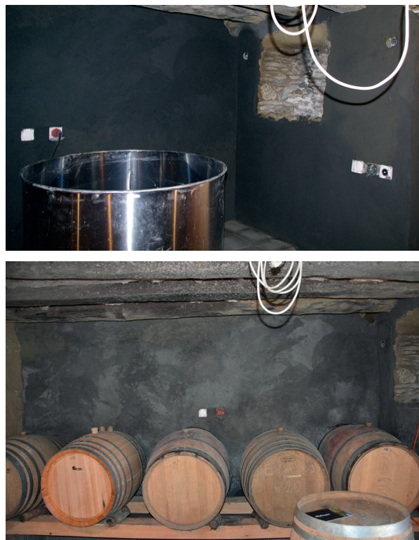
Figure 207 and 208. Different ratios of biochar, sand and clay create plasters with different colours. Pictures of the Ithaka Institute wine cellar.
