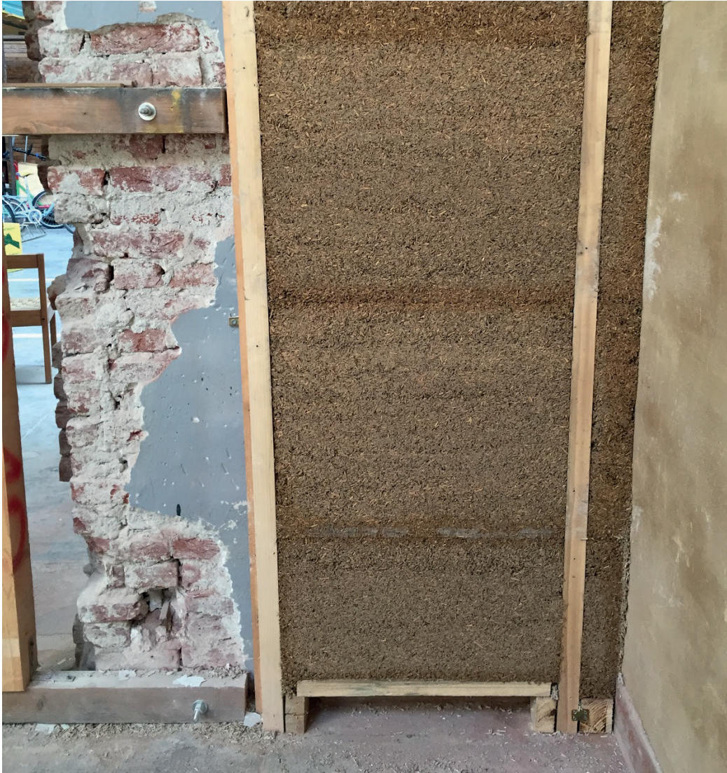
Figure 158. The hempcrete after the shutterings were taken off on the right side of the north wall. Photo Andi Dani
