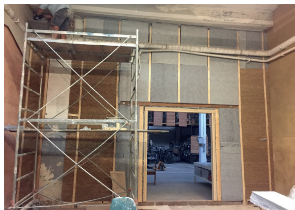
Figure 38. The south wall insulated using hempcrete and SNTHERM 40 100 insulation panels.
