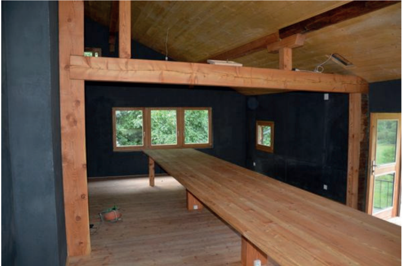
Figure 209. The biochar plaster applied on the walls of the indoor areas on the Ithaka Institute.
