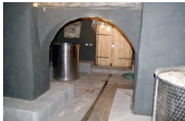
Figure 206. The Ithaka Institute wine cellar after the biochar plaster was applied and dried.
