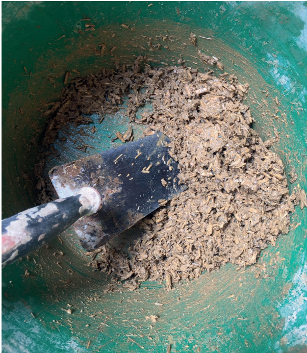
Figure 116. Earth from subsoil and hemp shiv being mixed with a trowel.
