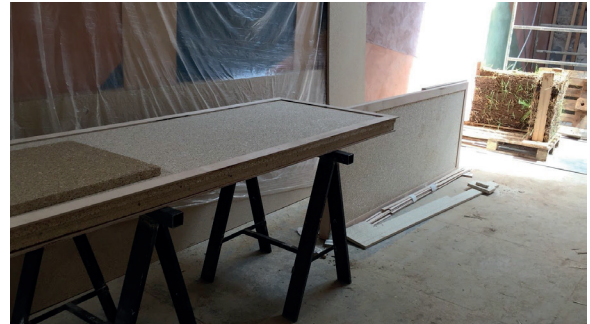
Figure 42. The hemp doors built with the CANAPALITHOS 350, timber and hemp fibers.
