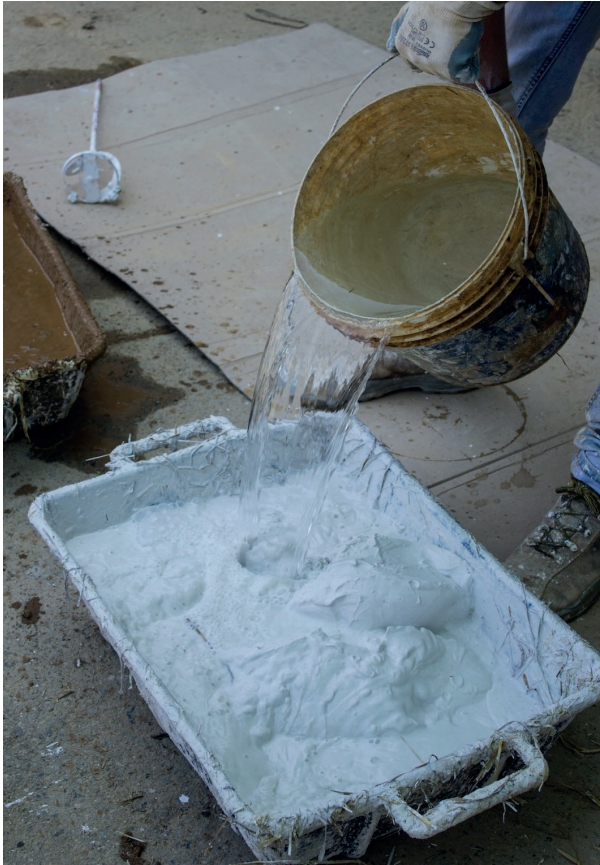
Figure 90. Water being added to the lime putty to prepare the lime slip.
