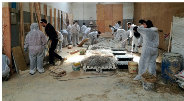
Figure 102. Students preparing of the lime straw mixture during the workshop of 23 May 2017.
