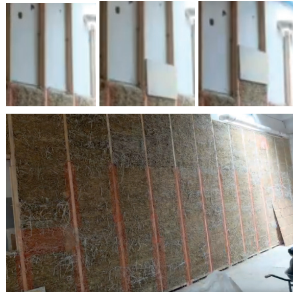
Figure 97, 98, 99 and 100. Top, the process of filling, going from bottom up, while using the same wooden board for the shuttering, and bottom, the insulated wall . Pictures extracted from the timelapse of the 26-29 May 2017 workshop
