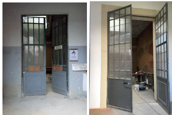
Figure 29 and 30. The entrance door before (left) and after (right) it was rotated and changing the glasing elements. CANAPALITHOS 350 were fixed around the door.
