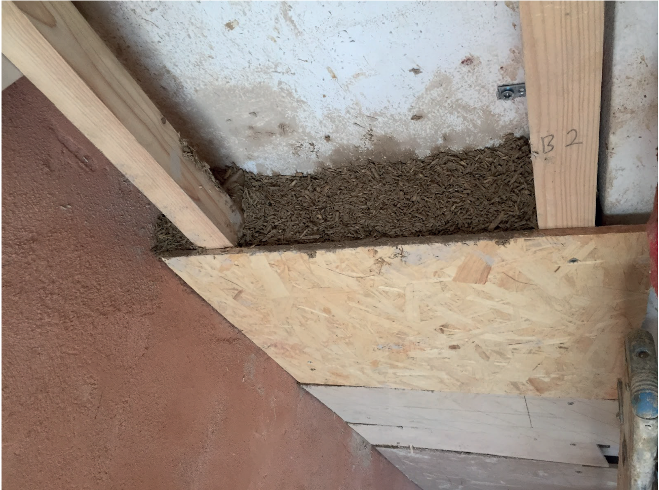
Figure 152. The hempcrete mix once cast and pressed inside the shutterings Photo: Andi Dani
