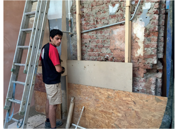
Figure 146. The timber frame and the shutterings created by different wooden boards. Photo: Andi Dani
