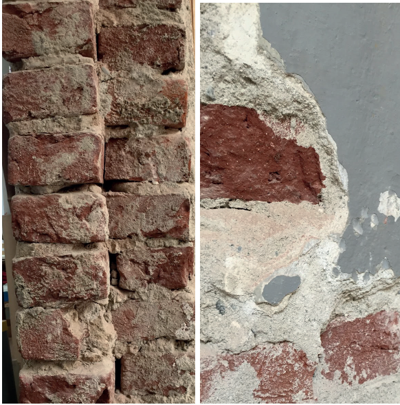
Figure 9 and 10. Double layer of solid bricks wall and the cement and sand plaster. Photos: Andi Dani
