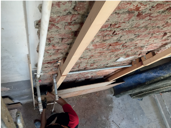
Figure 145. The 5x5 cm fir joists fixed against the wall. A 10 cm bedding is created by the addition of 5 cm timber spacers between the wall and the joists. Photo: Andi Dani
