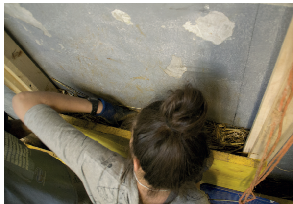
Figure 76. The filling process done manually, during the which a horizontal wooden batten was added every 25 -30 cm. Photo: Jasenko Spahic
