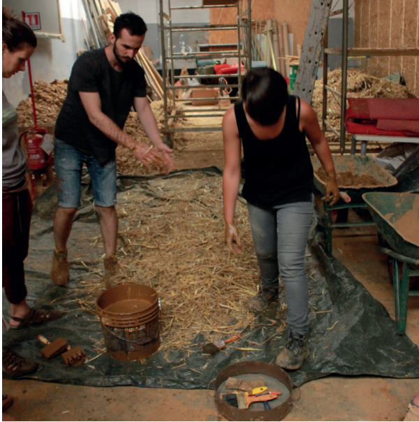
Figure 70. After the straw was spread over impermeable bags, the process of mixing took place, by gradually pouring clay slip over the straw and mixing it. Photo: Jasenko Spahic
