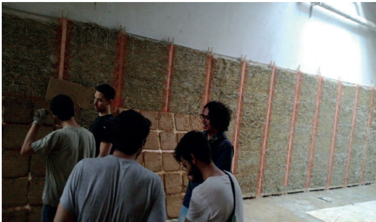
Figure 104. The bottom part of the eastern wall completely insulated. This portion of the insulated wall is 12 m long and 2.5 m high. It took around 6 hours for 20 students to complete this operation. This low productivity ( 0.25 \text{ m}^2/\text{h} ) was due to the lack of experience of the students, and the fact that the total number of the participants was 46 people, and they took turns on the different processes required for the insulation construction. A faster application time was obtained later by the more experienced students, and it reached 15\text{-}20 \text{ min}/\text{m}^2 .
