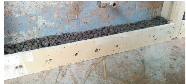
Figure 88. Expanded clay used to fill the space between floor and the light straw clay insulation in another spot of the room.
