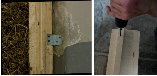
Figure 55 and 56. Left, the stud fixed against the wall using a steel L-shaped elements and screws, right, the process of fixing the wooden batten along the 10 cm side of the stud.
