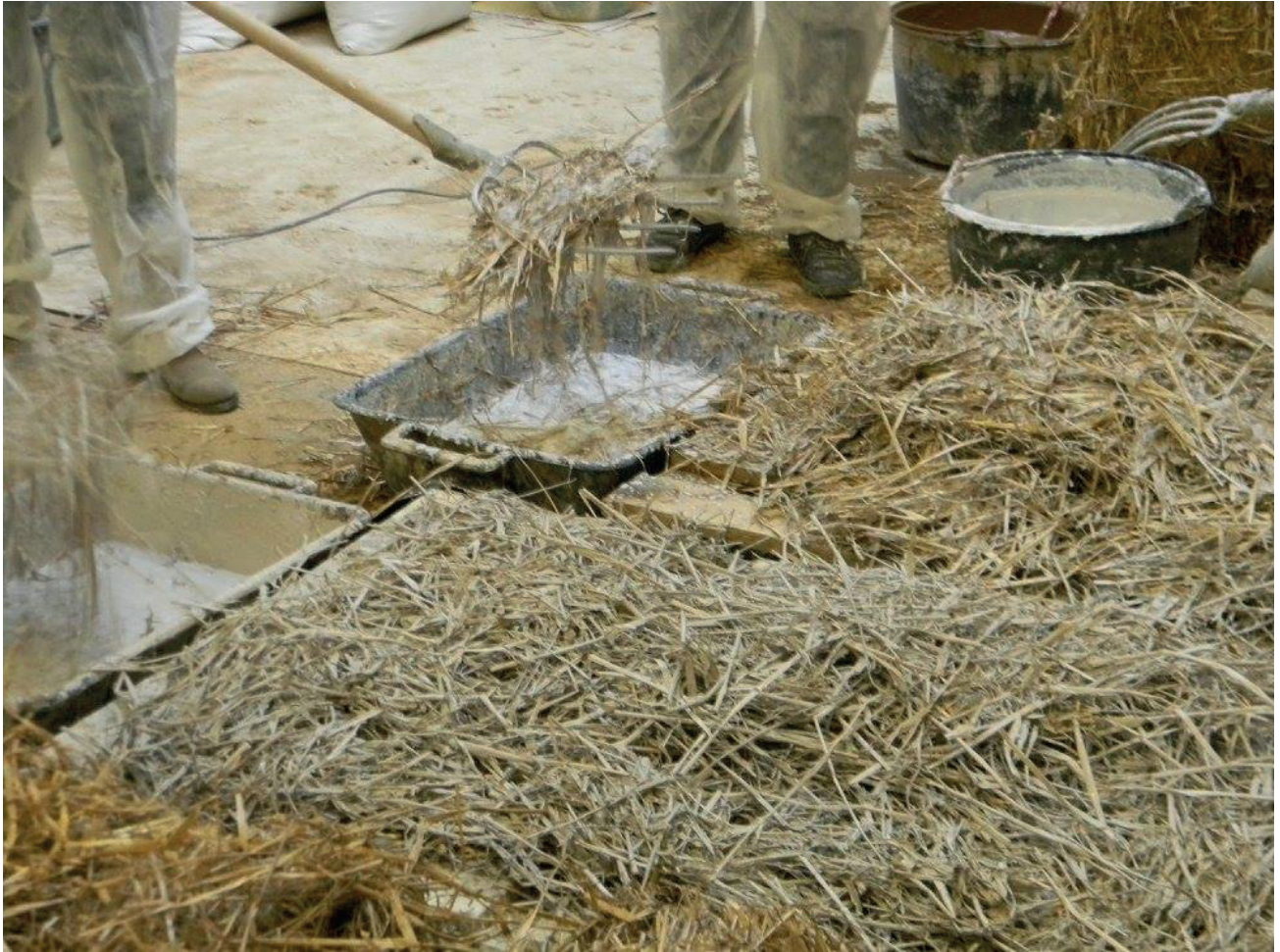
Figure 94. Straw being soaked and dripped in tanks filled with the lime putty slip. Photo: Stefano Iurlaro
