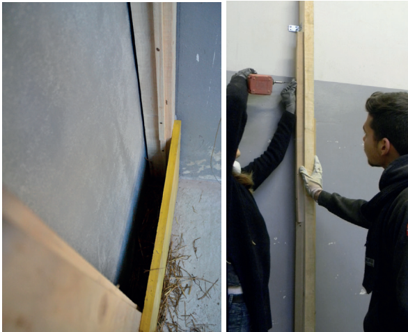
Figure 57 and 58. On the left, one shuttering completely finished and ready to be filled. On the right, two students fixing the wooden batten to the upright.
