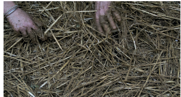
Pictures 72, 73 and 74. Straw and clay slip getting manually mixed.
