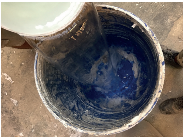
Figure 147. The first step: 18 litres of water being poured inside a barrel.
