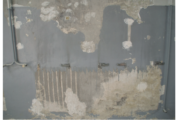
Figure 12. Degraded plaster and painting in the Red Room. Photo: Arthur Bohn
