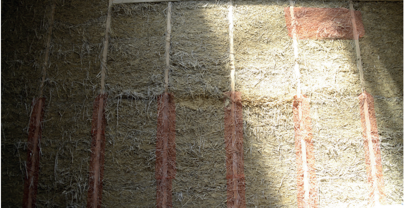
Figure 86. Part of the eastern wall after the application of the lime straw insulation.
