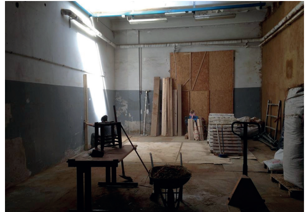
Figure 15. Picture showing the wall that divides the Red Room from the “Officine Creative”. The wooden boards at the center of the wall are covering a void where there used to be a door that connected the two areas.
