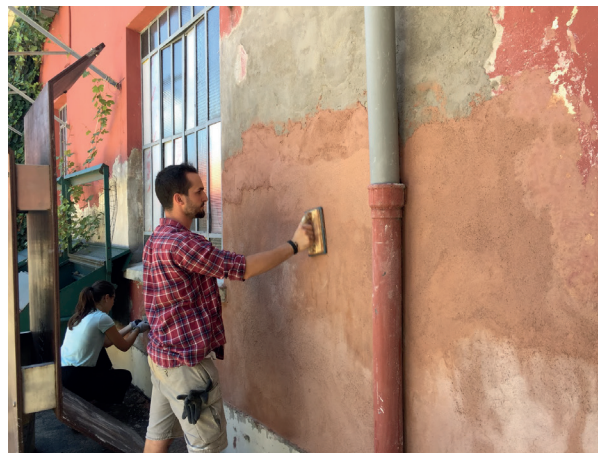
Figure 31. The cocciopesto plaster being applied on the facade wall of the Red Room.
