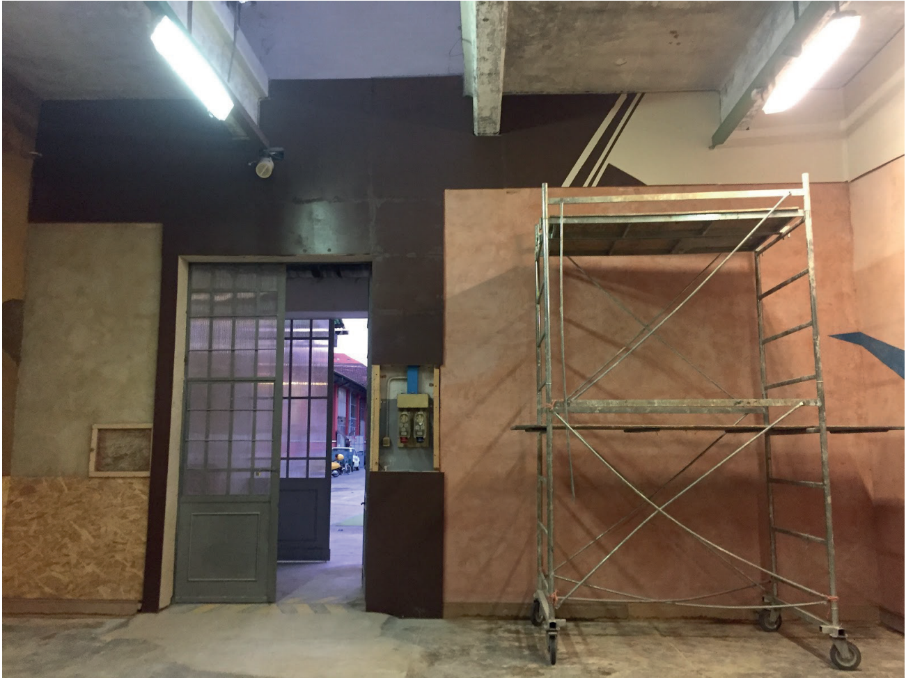
Figure 37. The entrance and part of the east wall after the insulation panels made of recycled plastic were applied, covered with birch wooden boards and painted during the second phase.
