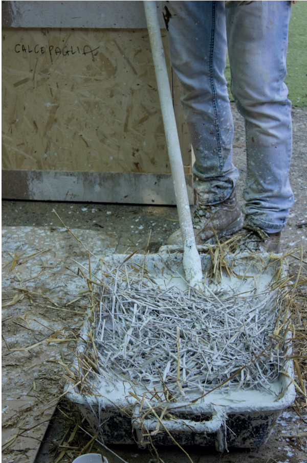
Figure 95. The soaking of the rice straw in the lime slip. It can be seen the excessive amount of humid binder around the straw stems, which brought to the decision of mixing the soaked straw with additional dry straw in order to create a mix with an adequate density. Photo: Jasenko Spahic
