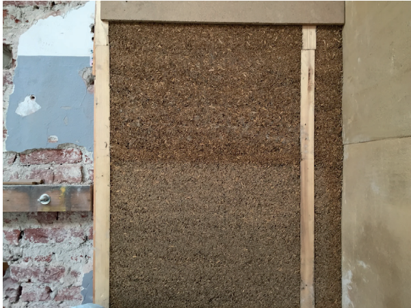
Figure 153. The shutterings on the left side of the wall were taken off several days after the mix was cast. The colour difference is due to the use of different shuttering boards, MDF panel above and impermeable fiberboards below (still wet).
