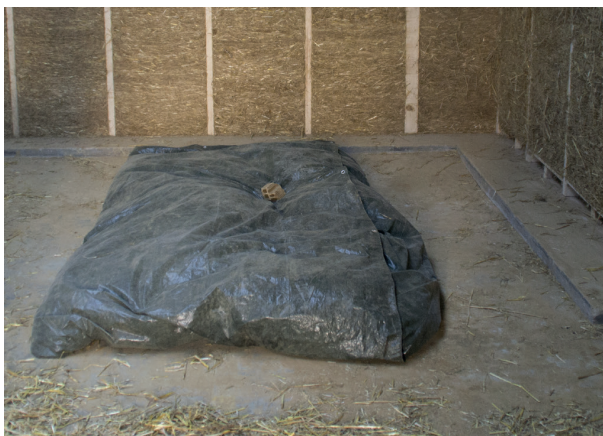
Figure 75. After the mixing process is finished, the composite material is left from 2 to 12 hours to rest in a dry spot, covered by an impermeable bags. Photo: Jasenko Spahic
