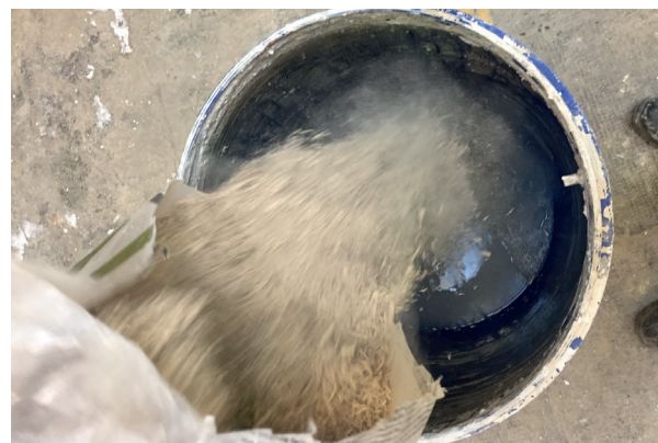
Figure 148. The second step: one full sack of premixed hemp shiv and binder (CANAPAMAS 385) is added to the water.
