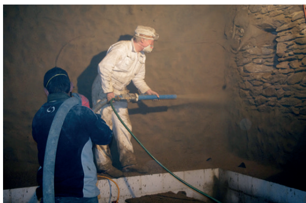
Figure 205. Biochar plaster applied with a spraying hose in the wine cellar of the Ithaka Institute, Switzerland.
