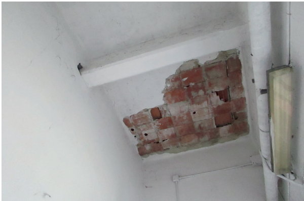
Figure 11. The paint and the plaster have fallen of in the entrance room, revealing roof slab made out of perforated bricks. Photo: Andi Dani
