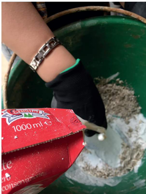
Figure 129. Milk being added to the lime putty-hemp shiv mixture, while constantly being mixed with a trowel. Photo: Andi Dani
