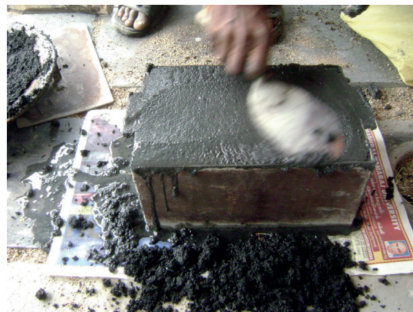
Figure 220 and 221. The composite produced by mixing biochar, sand and cement is poured gradually in the form, while constantly pressing the mix in order to obtain a compressed brick. Source: http://e-biocharbricks.blogspot.com/
