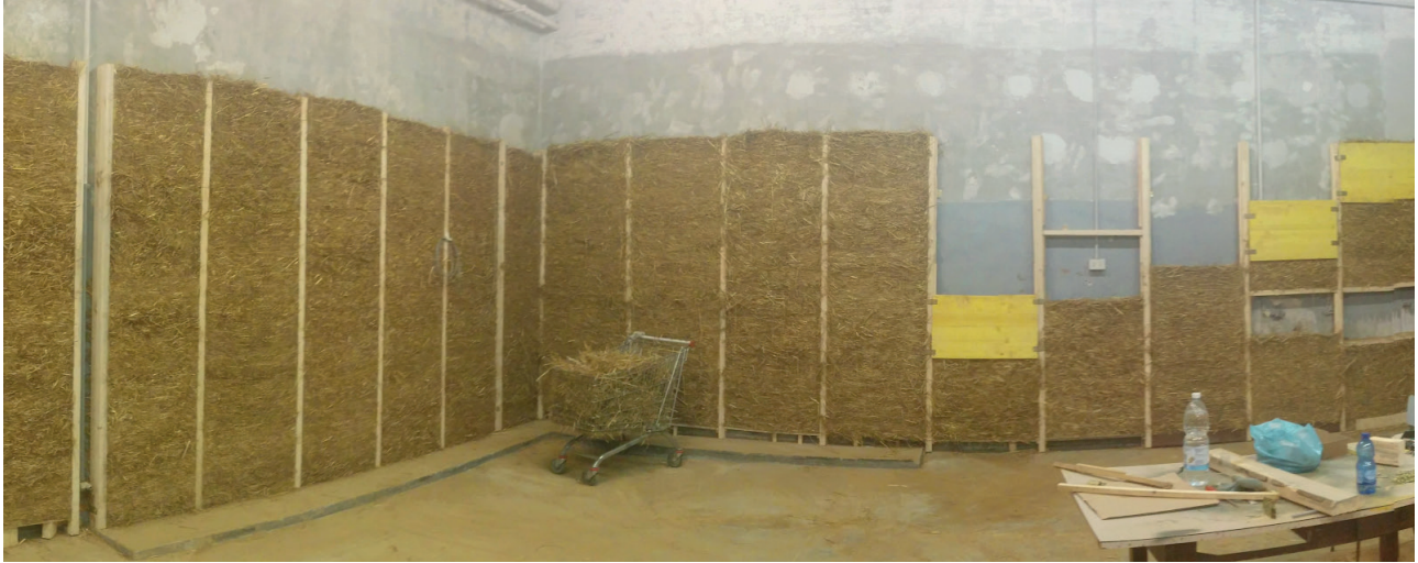
Figure 78. Straw and clay insulation as applied in the Red Room. The northern wall is in the front view. Photo: Nicoletta Palama
