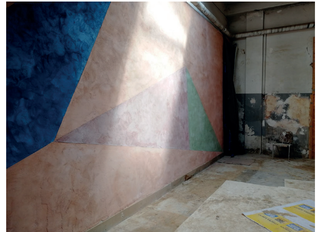
Figure 27. The eastern wall after the straw-lime implementation and plaster application Photo: Angelo Iurlaro
