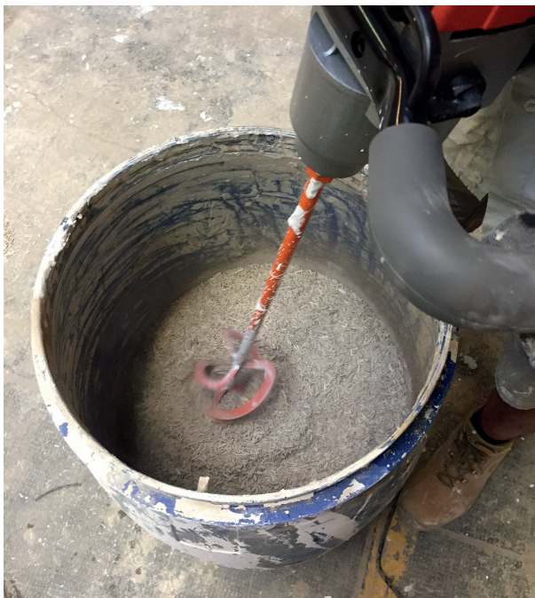
Figure 149. The third step: mixing the biocomposite using a drill mixer.
