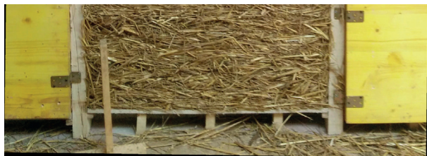
Figure 62. Light earth insulation applied and wooden board taken off showing a way to detach the insulation from the floor.
