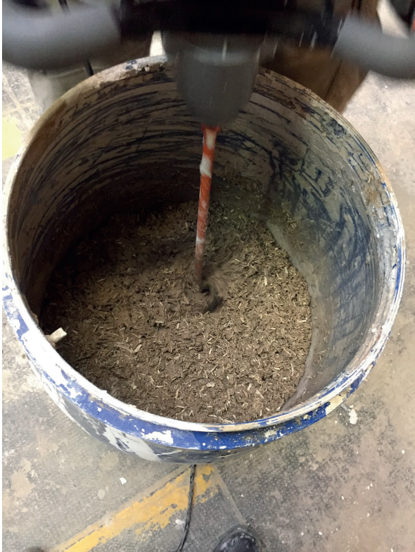
Figure 150. Hempcrete getting mixed with a drill mixer becoming homogeneously saturated. Photo: Andi Dani
