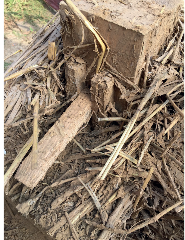
Figure 59. The jointing system between the vertical battens and the horizontal wooden element, if the light earth is used as an infill material in a free-standing wall. In our case there was only one vertical wooden batten, because the wall would serve as a support from the other side.
