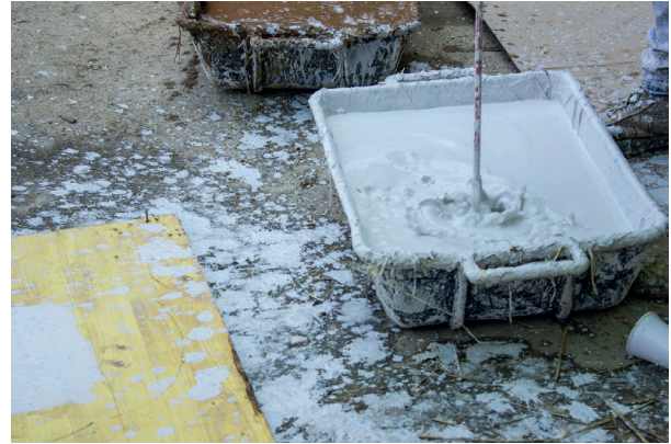
Figure 91. The lime putty and water being mixed by an electrical mixer in order to get a more homogeneous slip.
