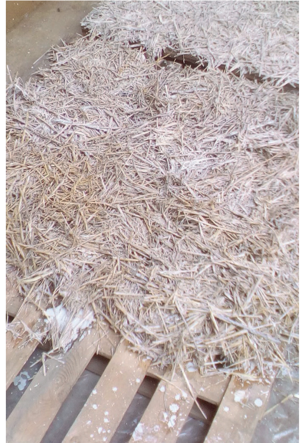
Figure 96. Soaked straw laying on wooden pallets is let to drain for a short period of time before being cast in the shutterings.
