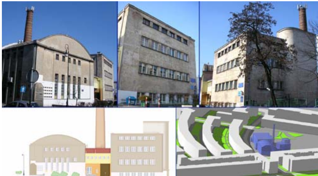
VI Colony: the former heating plant and ex-laundry. Survey and 3D representation of the area
