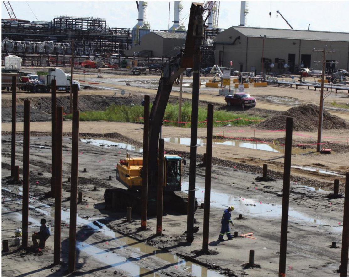
Fig. 2 Typical helical pile installation (from Sakr, 2015).
