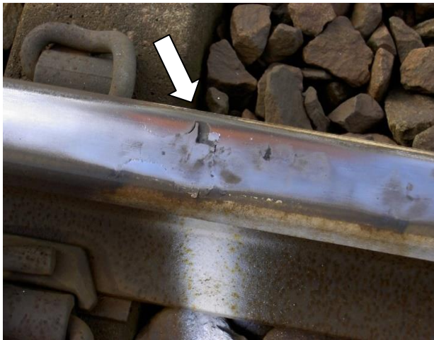
Figure 9: The error is verified and marked with white color on the outside of the rail.
