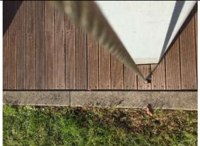
Figure 98 Columns serve as the element which supports the cable that is anchored in the ground.
