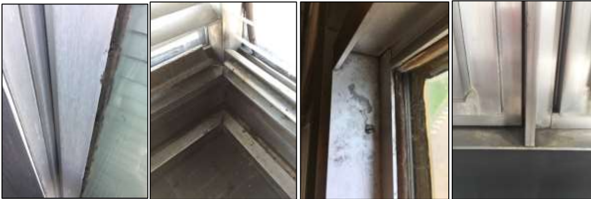
Figure 44 Representation of the damages and degradation due to the leakage and harsh weather conditions.
