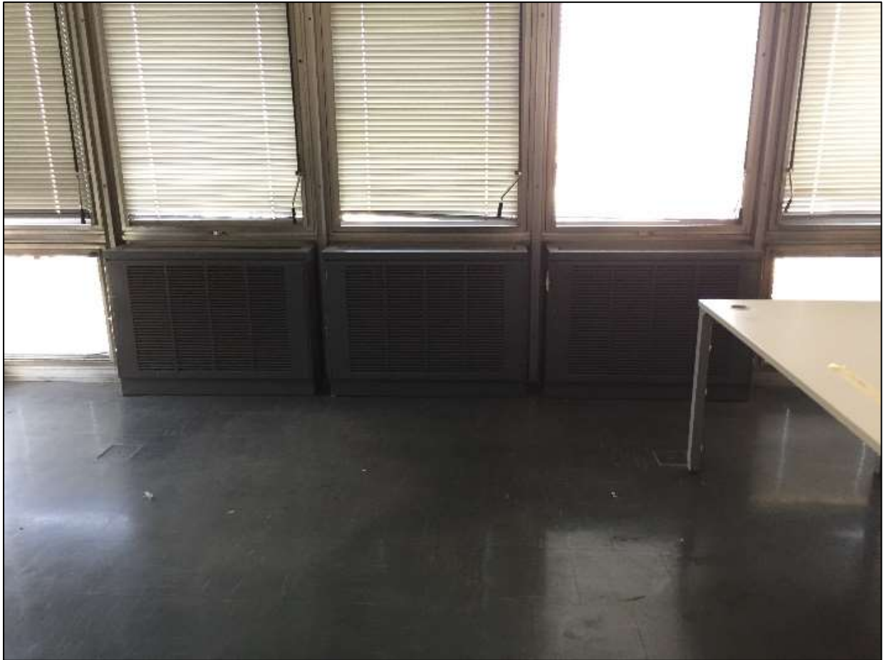
Figure 40 The fancoil units
