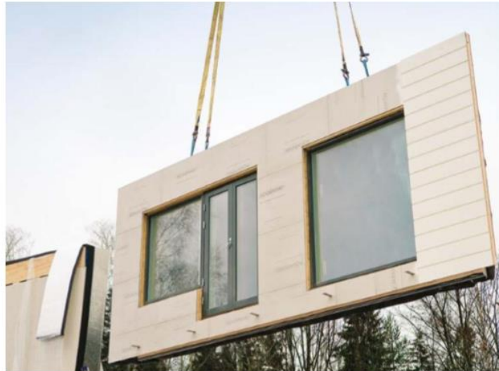
Figure 4.2 - Example of XLAM panel [17]
