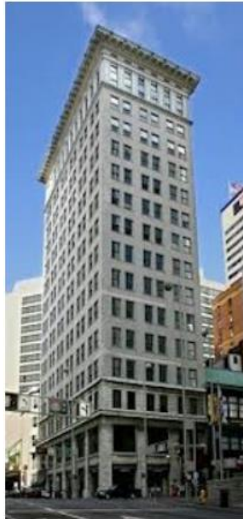
Figure 3.1 - The Ingalls Building in Cincinnati, Ohio [15]
