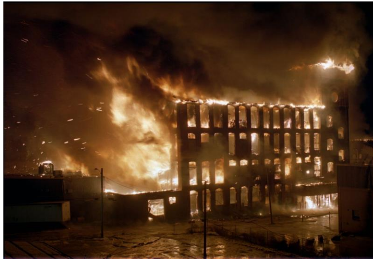
Figura 3.4 incendio Malden Mills 1955
