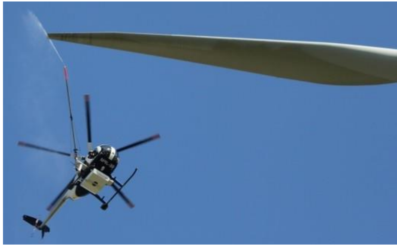
Figure 1.14. Manual de-icing of a wind turbine [24]
