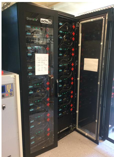
**(a)** 25 kW / 25 kWh Lithium-Titanate battery: The 13 modules can be clearly distinguished and easily accessible.
