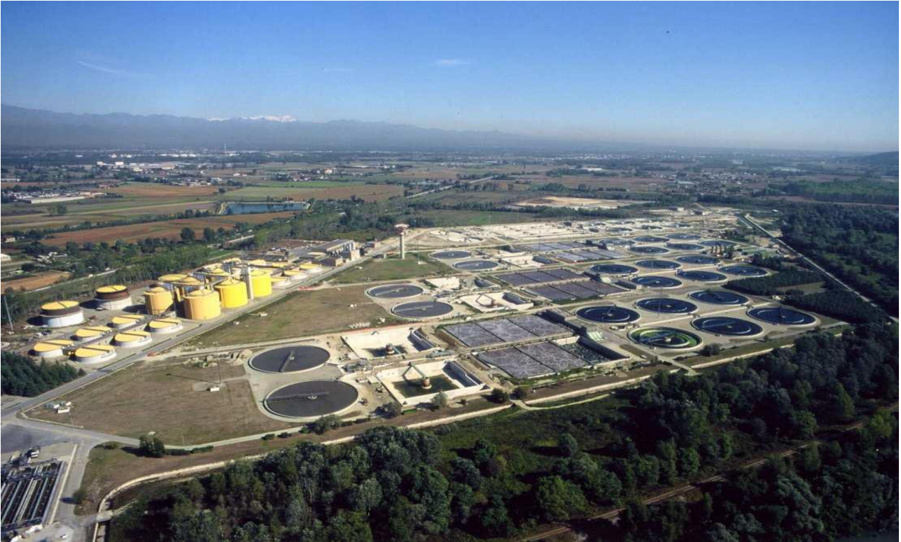
Figure 1: Castiglione Torinese waste water treatment plant.
