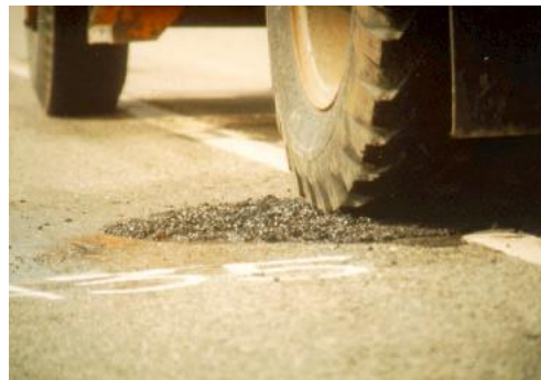
Figure 2.4: Throw-and-roll procedure, patch compaction - Wilson P & Romine R, 2001
