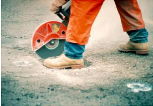
Figure 2.7: Semi-permanent procedure, edge cutting - Wilson P & Romine R, 2001
