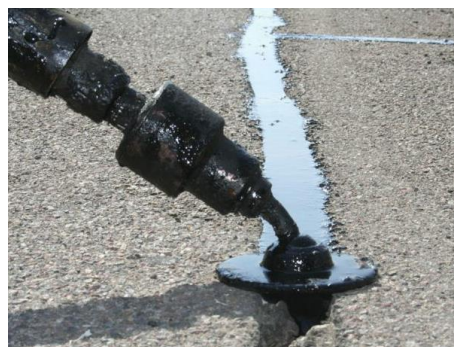
Figure 2.6: Edge sealing procedure, AsphaltPro
