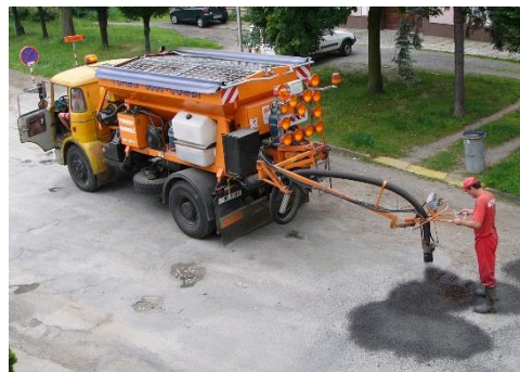
Figure 2.10: Spray-injection device, truck mounted unit - Michal Mañas
