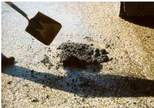
Figure 2.3: Throw-and-roll procedure, material placing - Wilson P & Romine R, 2001
