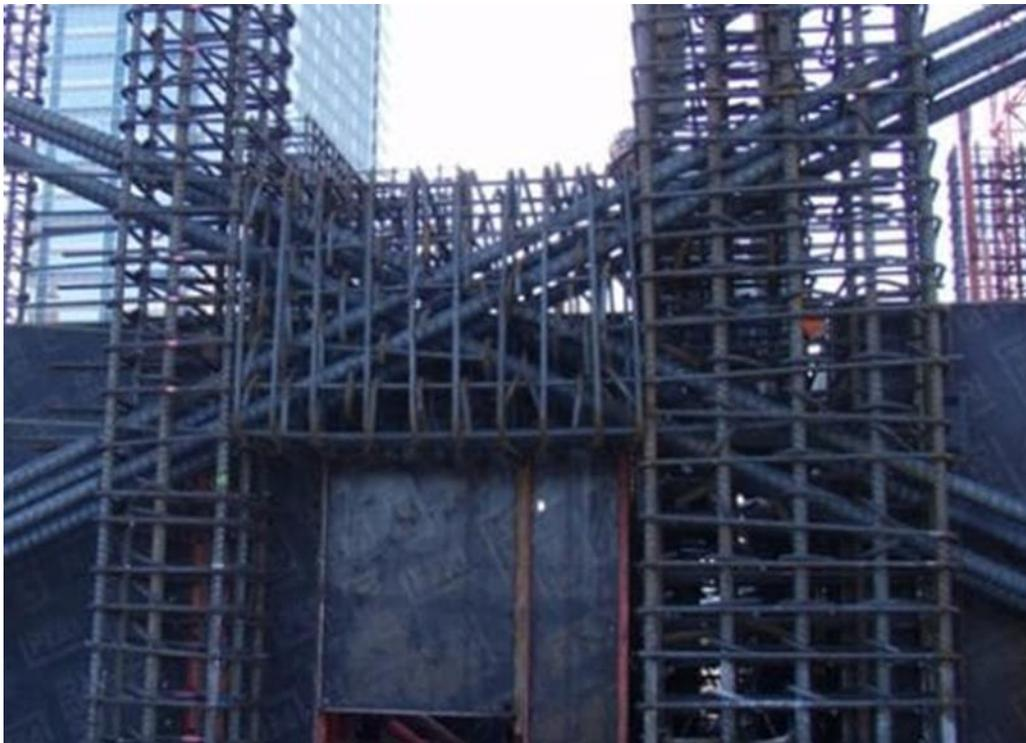
*Figure 4.13 Example of Diagonally Reinforced Coupling Beams*
