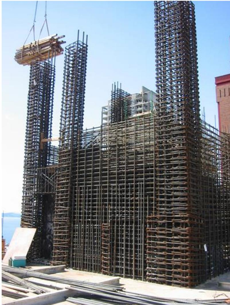
*Figure 4.9 Example of Shear Walls Reinforcement*
