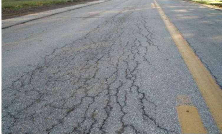
Figure II-11. Fatigue Cracking
