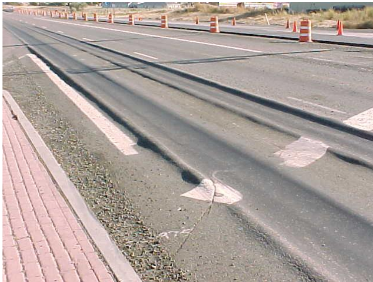
Figure II-10. Rutting
