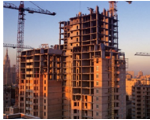
Contemporary house blocks
