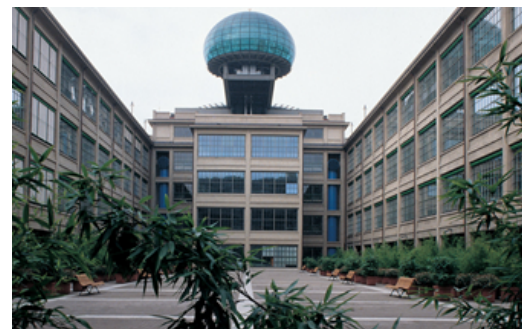
Lingotto, internal courtyard
