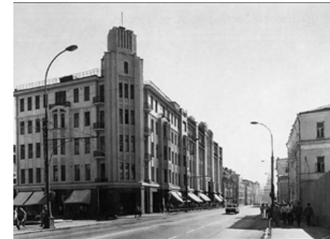
Voentorg, exterior view Original building
