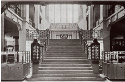
Voentorg, interior view Original building
