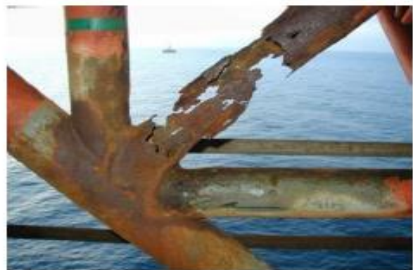
(B) Corrosion
