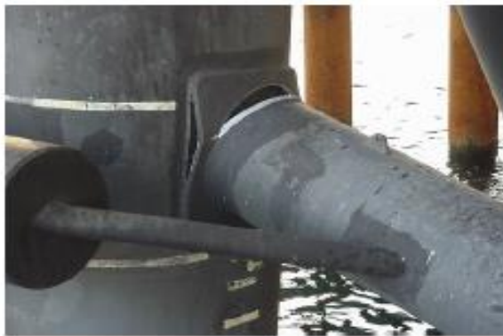
(A) Fatigue through crack
