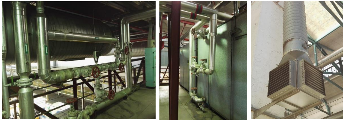
Figure 27 - Photos of CTV number 3: on the left the bypass system and electrical panel with carry comands, on the right the pipeline to fed the battery. The last photo is the last part of the emission system called “testa di moro”.
