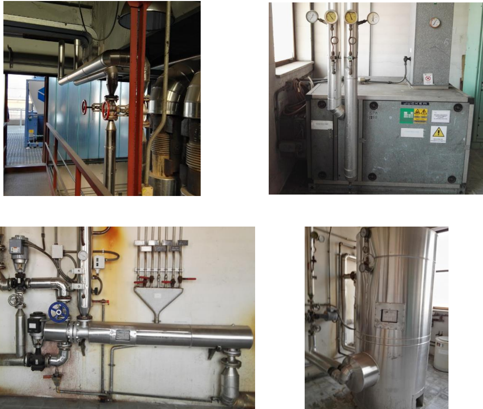
Figure 28 – HVAC in Control Unit of Dressing Rooms. Top left: Switch valve; Top right: CTV of Dressing Rooms; Bottom left: Heat Exchanger 140 kW; Bottom right: Boiler ACS
