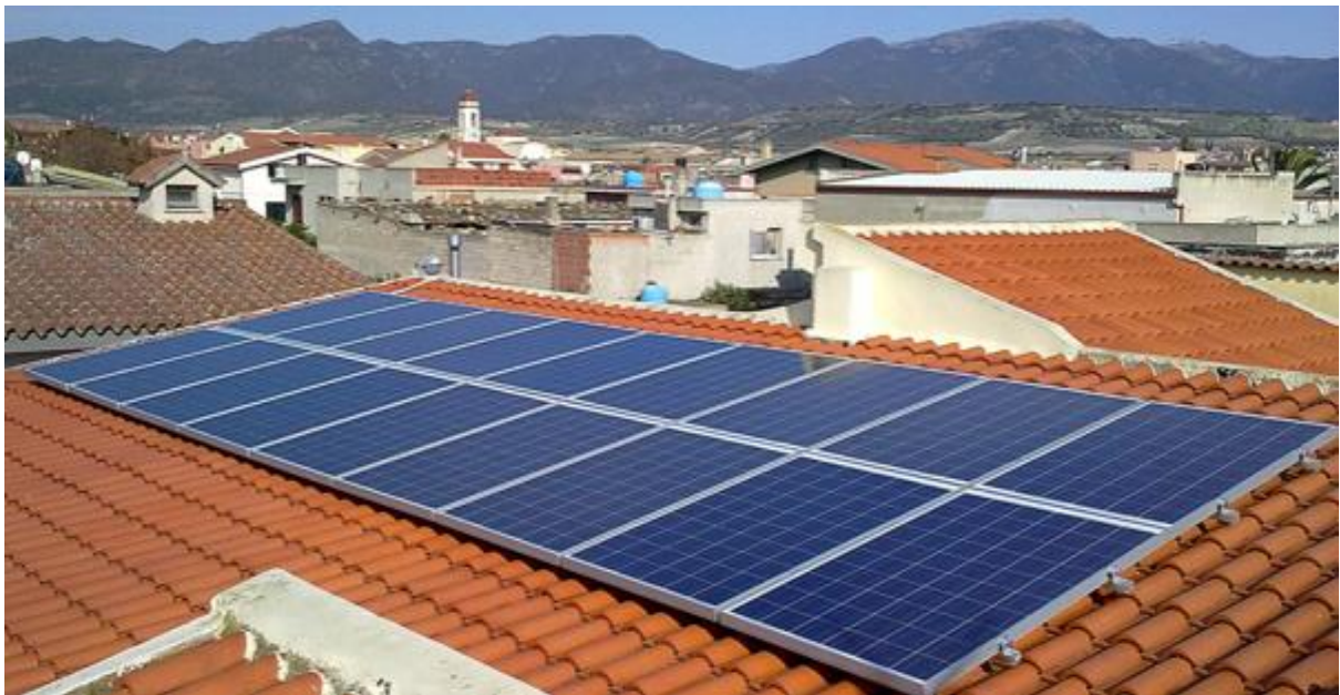
Figure 4.1: Polycrystalline PV modules installed on a household roof
