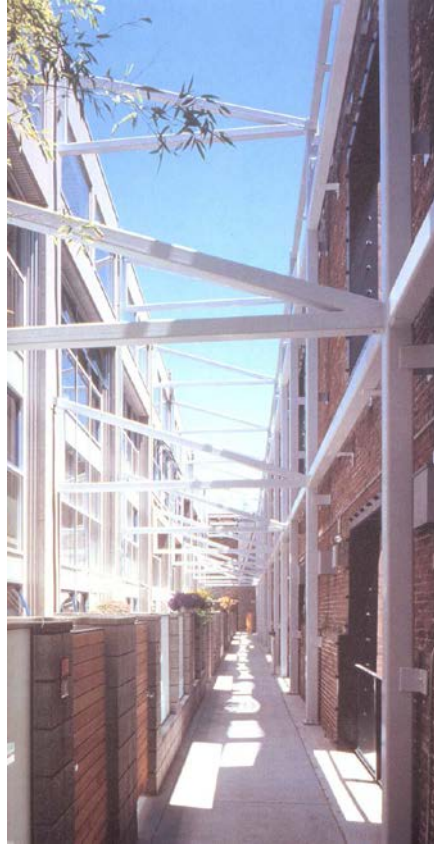
Structural elements were added to strengthen the old façade
