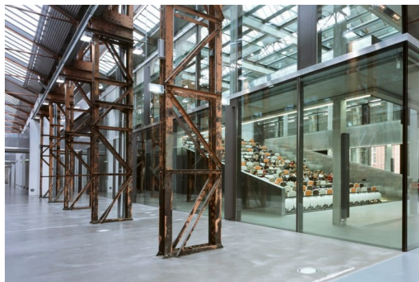
Thermal buffer zone between the new and old volumes
