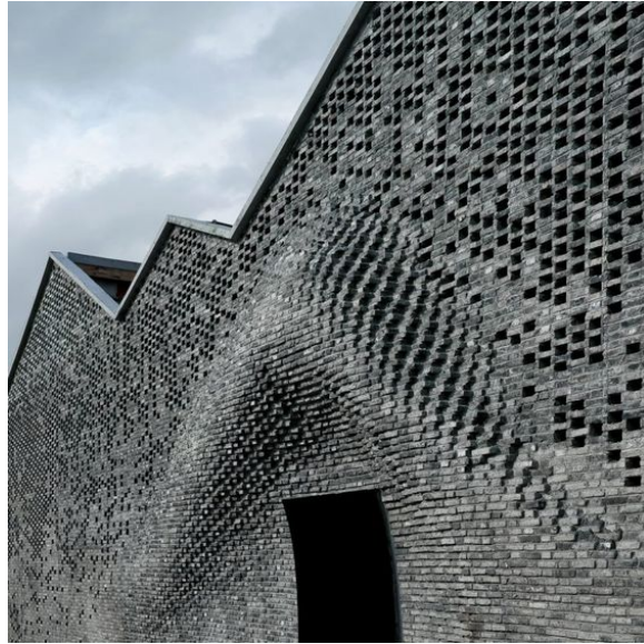
Chinese studio Archi-Union Architects programmed robots to construct the undulating brick facade of this art gallery in Shanghai's West Bund district.
