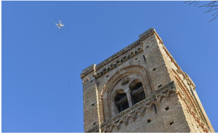
UAV Survey of the bell tower of Duomo Vecchio di San Severino Marche (MC), carried out using a DJI "Phantom 4 PRO" drone.
