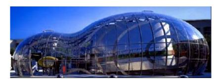
Figures show the Bubble Pavilion, Frankfurt 1999. The architect Bernard Franken and the structural engineers Bollinger+Grohman designed this freeform by using a glass-covered ribs frame. One of the main goals of this case study is to demonstrate that bar structures are suitable as structural systems in Blob architecture. The permeability to light has been the main requirement considered during structural and shape designing of the building
