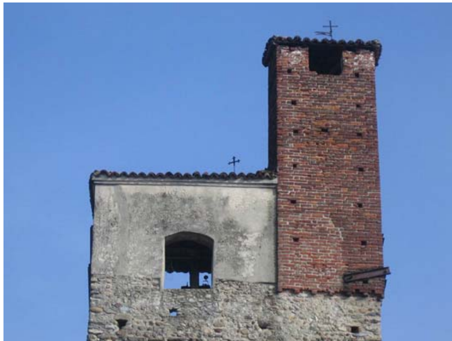
Front view of the typical watch-tower, the only preserved example in the whole Canavese zone
