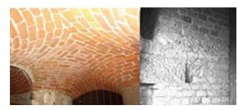
Two examples of the most important architectonic and constructive techniques: the "funnel vault" or "fungus vault", perfectly adaptable to the "Antonelli's system", and stone put into the brick wall (Sabrina Fassi)
