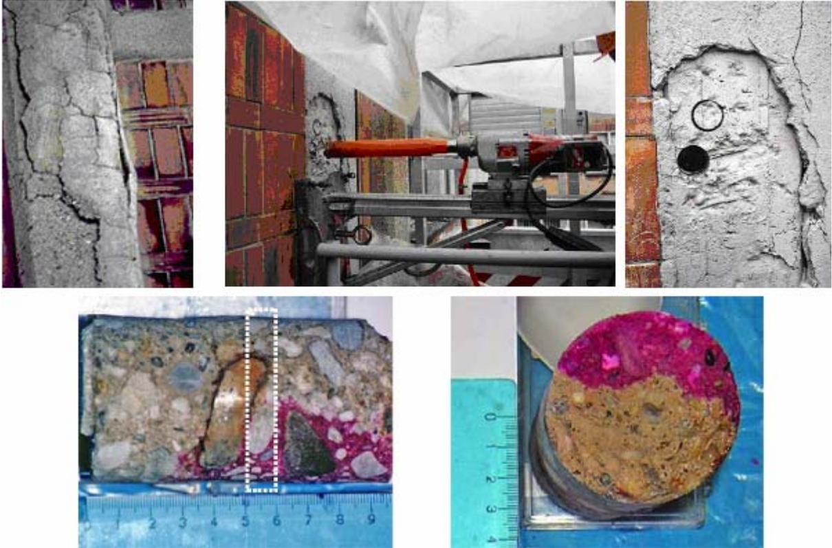
Therapy considers restoration techniques when concrete has suffered carbonation and iron rods have been oxidized causing cracks and spalling of the external concrete: realkalization, use of silanes, removal of carbonated concrete and restoration with fibre-reinforced at contrasted expansion grout.
