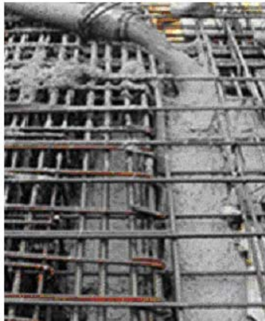
Filling of structure heavily congested with SCC.
