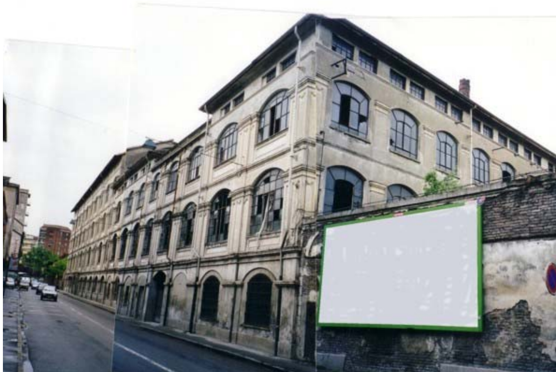
Paracchi's Carpet's Factory's façade on Pianeza Street in Turin.
