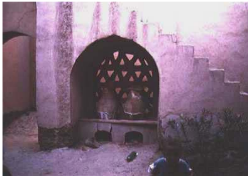
Fig. 3 Resthouse, building for climatic relieves, in New Gorna village. The building is built around a courtyard, furnished with vegetation and water jars, put inside the mazeer. All these systems co-operate to improve the internal microclimate.
