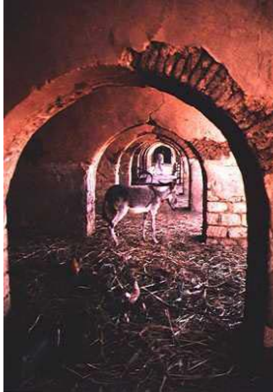
Fig. 2 New Gorna village, Luxor, Egypt. Covered area of the market, built with nubian vaults in earth bricks. Today the market is abandoned and is utilised just as dust place and stable.
