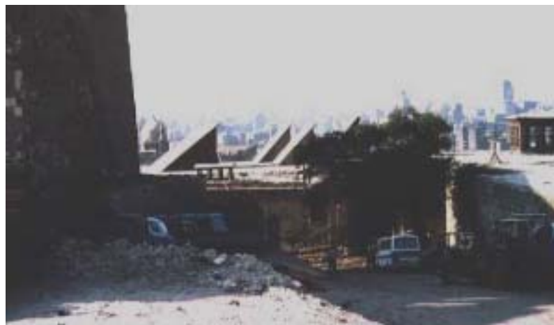
Fig.1 Malquaf, or wind-tower, seen from Cairo Citadel. The malqaf, facing north, receives the cool winds and avoids the direct solar radiation to enter inside the courtyards or the rooms, covered by that system.
