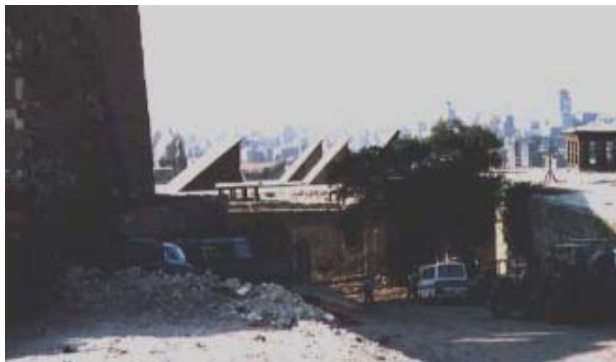
Fig.1 Malquaf, or wind-tower, seen from Cairo Citadel. The malqaf, facing north, receives the cool winds and avoids the direct solar radiation to enter inside the courtyards or the rooms, covered by that system.
