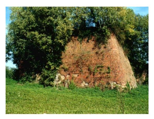
At the same time the walls will be cleaned and detached bricks put back. Afterwards the structure will be reinforced using ethyl-silicate and the walls finally cleaned. The diagnostics surveys will be now possible, no more hampered by self-vegetation, and it will be finally possible to restore the structure and proceed with final reinforcement and protection.
