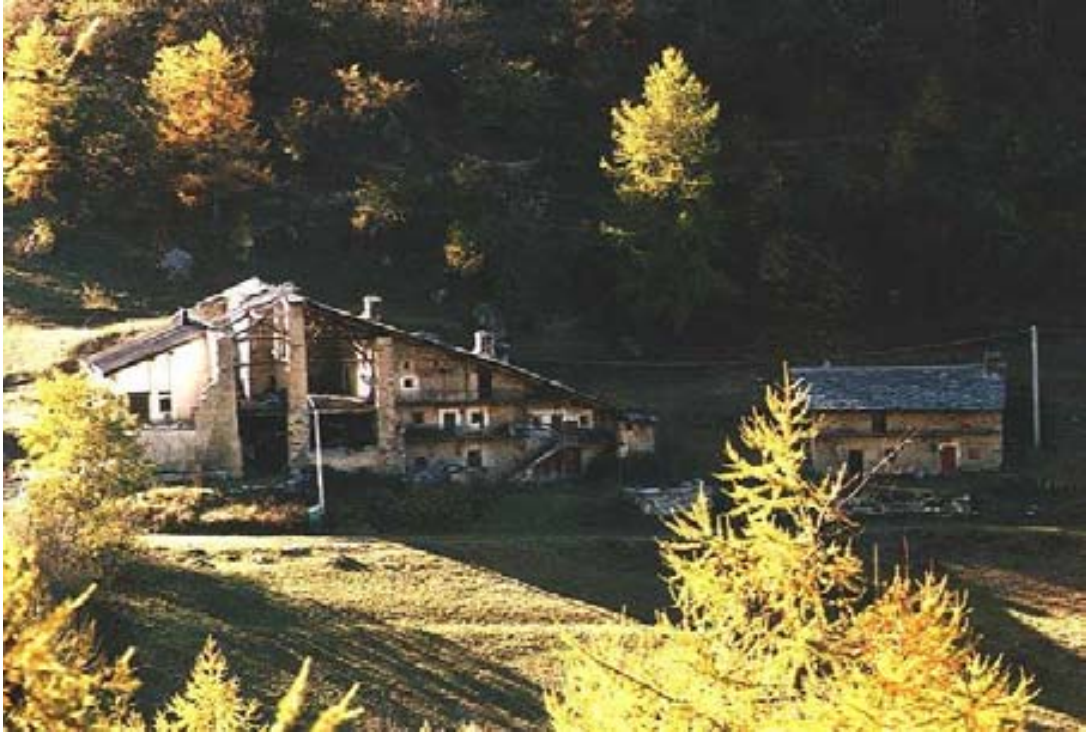
Casa Corte: overall view
