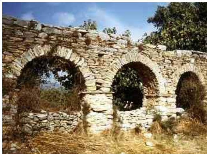
IASOS – Aqueduct – Flat stone facing. Opus alla Cilicia
