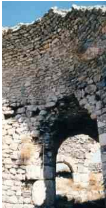
MILETO - Capito Baths – Laconicum dome. It's built by radial stone disposition
