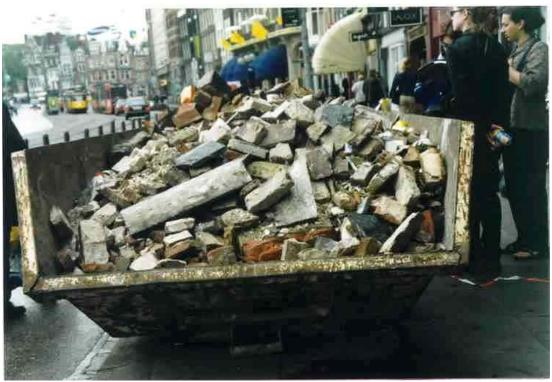
Conteiner for the distribution of the different fractions of construction or demolition waste
