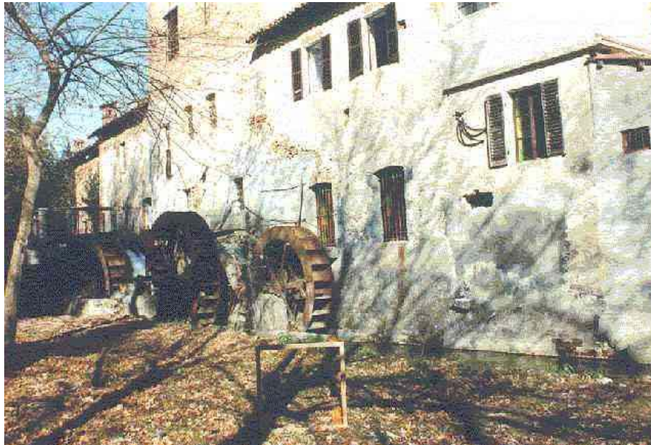
The Pogliola's water mill
