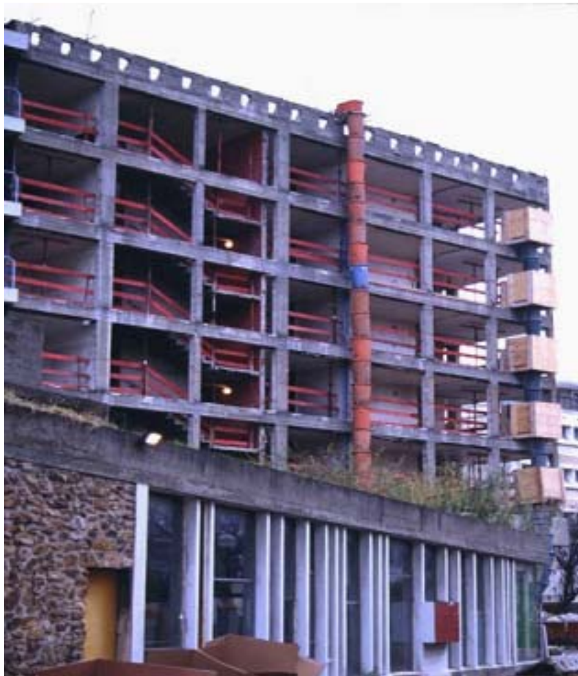
Demolition of the walls of the west facade. December 1999
