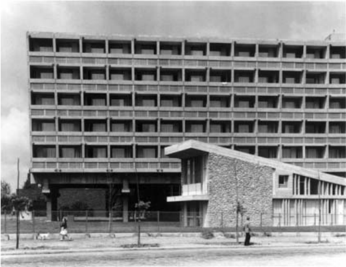
East facade at the end of construction. June 1959. FLC L 2 643
