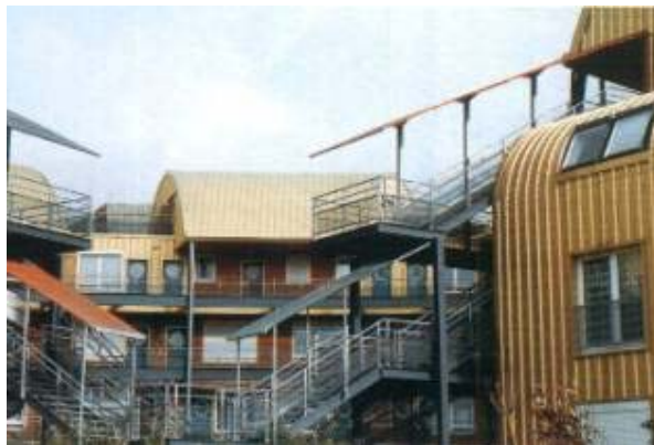
PICTURE 1 – Dry assembled building: Kronos in Nantes (Arch. Dubosc e Landowski)
