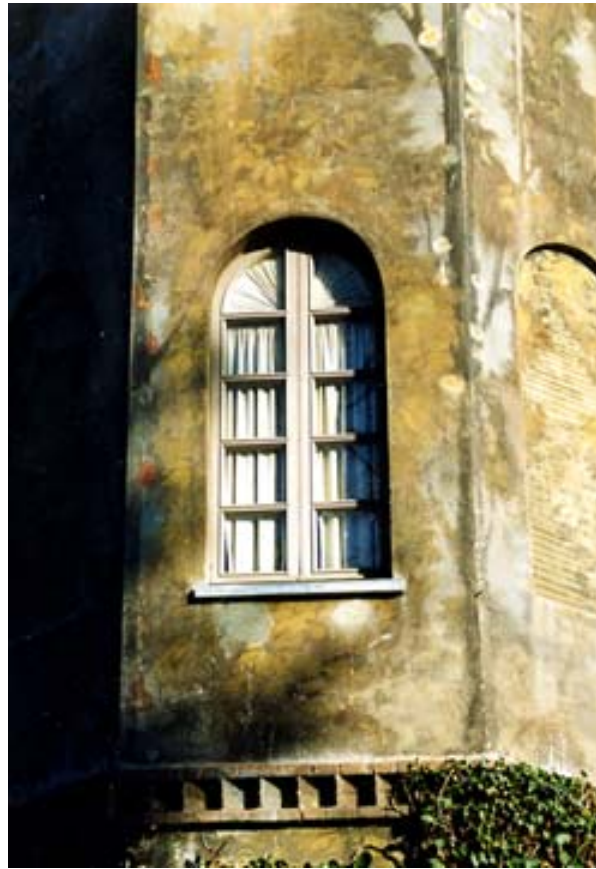
Detail of painted plaster on octagonal tower
