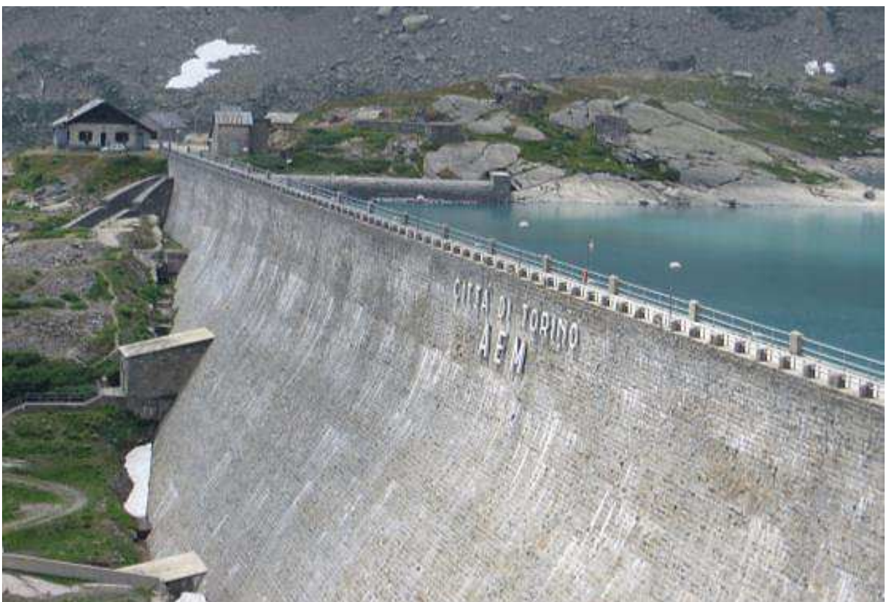
Orco Valley - The Serrù Dam (2015)
