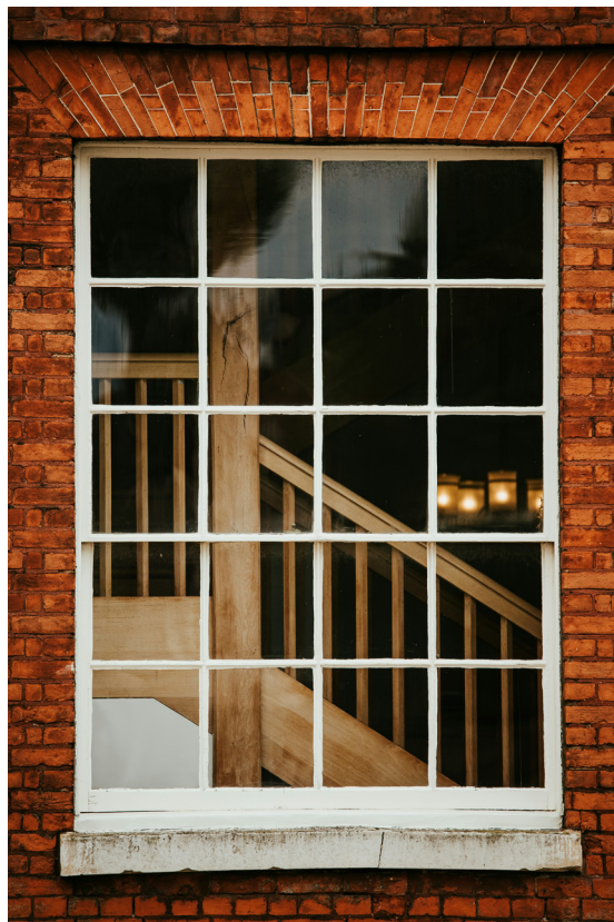
Figure 31. Window with single-pane glass and thin frame. [86]
