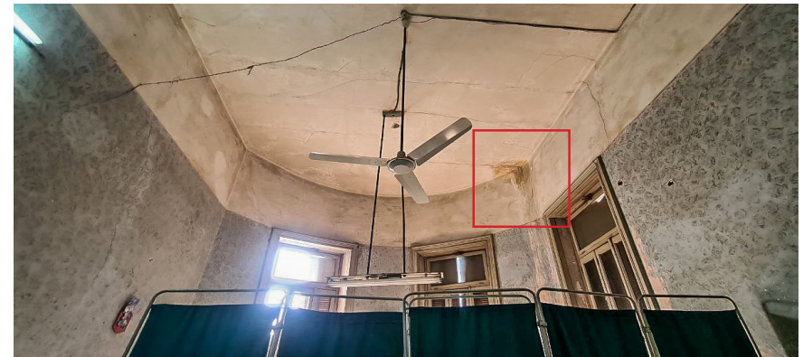
Figure 4.96 Interior of the medical clinic on the first floor, showing water leakage and poor condition. Photo by the author, December 2024.
