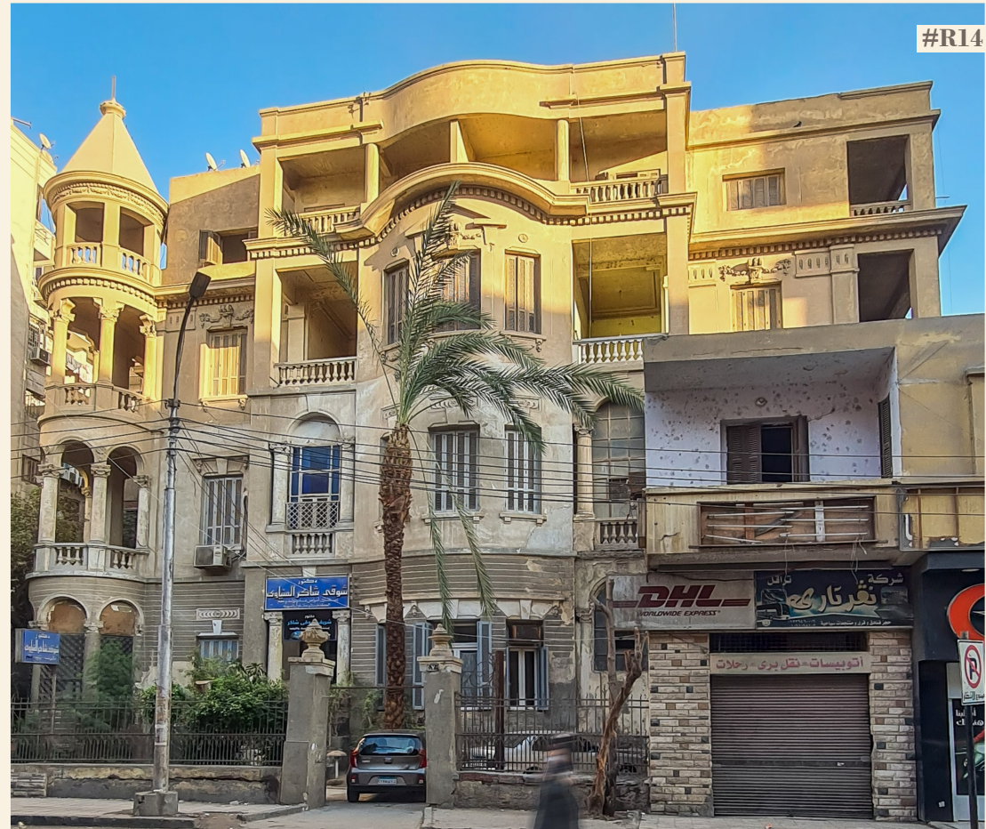
#R14-Building No. 7 ( Adel EL Minyawy palace), located on Al Gomhorya Street, is designed in the Beaux-Arts style. It is in good condition overall but requires maintenance, particularly for the balconies, where some leakage is visible on the façade. The building was officially registered in 2009 and currently serves residential purposes, with administrative functions on the ground floor. In the garden, a newer two-story structure serves both residential and commercial uses. The photograph was taken by the author in September 2025.
