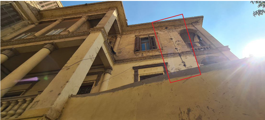
Figure 4.95 Facade view, showing the removed rainwater drainage pipe. Photo by the author, December 2024.
