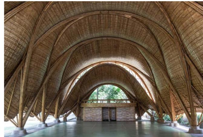
Figura 77. "Bamboo Structre of the Arc at Green School Bali". Photo: Tommaso Riva. <https://archello.com/it/news/dettaglio-struttura-in-bambu-dell'arco-della-green-school-di-bali>
