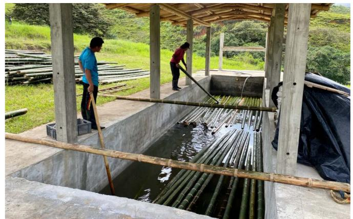
Figura 64. "Adding bamboo poles to our treatment tank".
