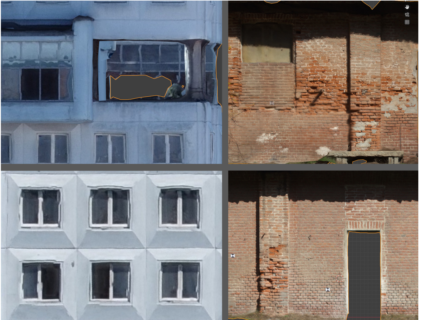
Figure 33. Comparison of photogrammetry results: House of Soviets (left) and Stupinigi Stables (right). Source: Ivan Karnitckii, Restoration and integrated conservation B, 2024.
