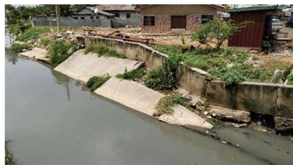
Figure 5.17: NIMA Drainage Channels in deteriorated condition (source: GARID)
