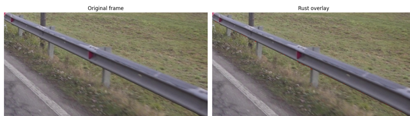
Figure 4.17: Example of how retroreflectors don't affect corrosion estimation.
