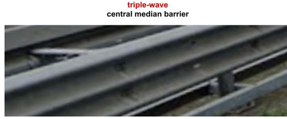
Figure 5.4: Example of the most frequent classification error on Google Street View data: the lower portion of a central median barrier is partially occluded or removed by the segmentation, leading the classifier to assign the ROI to the triple-wave class.
