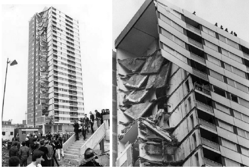
Figure 1 – The Ronan Point apartment building collapse, London 1968
