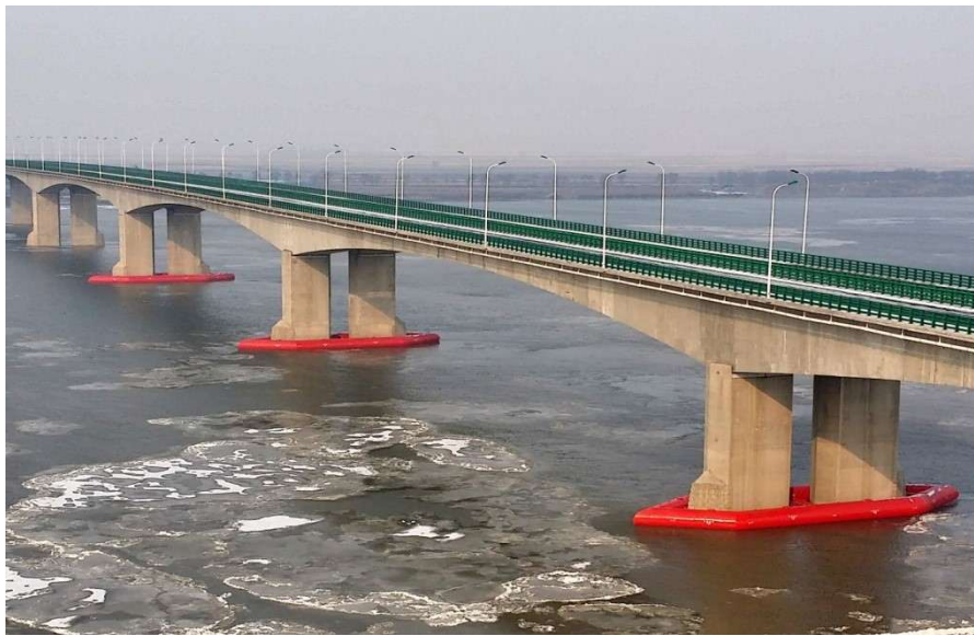
Figure 6 – Anti-collision devices for bridge piers
