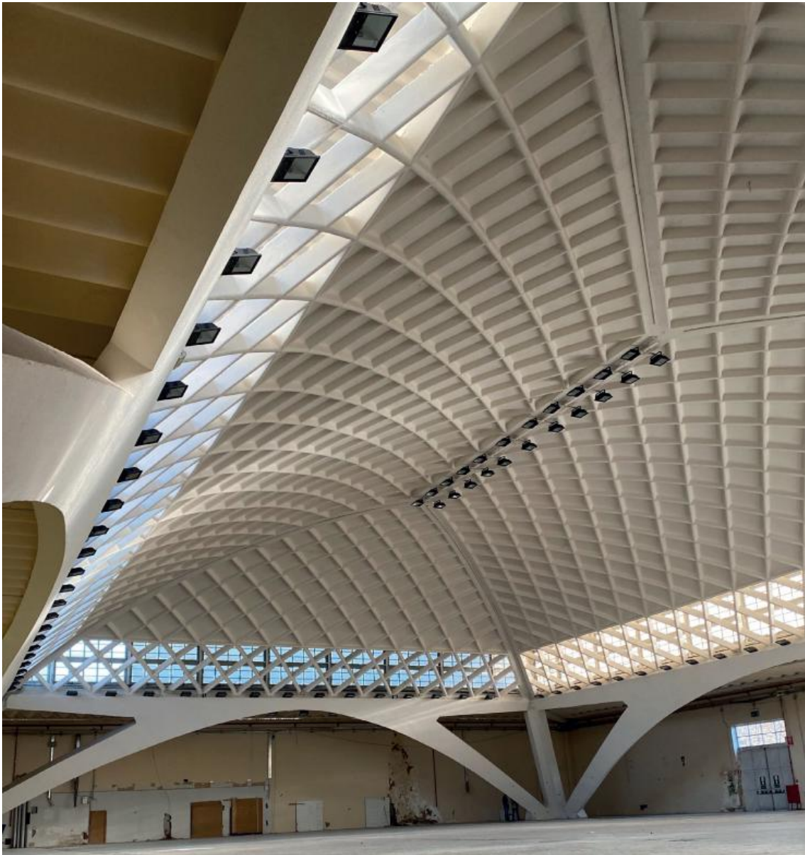
Figure 3.1 Hall C in Torino Expositions, the inclined arches and the ribbed ferrocement vault.
