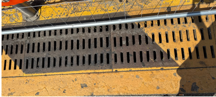
Figure 2.12: Collector channel located inside the parking lot
