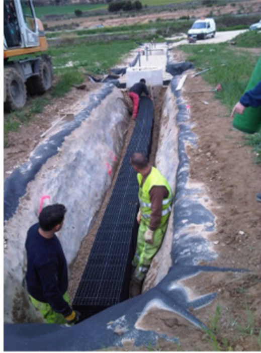
Figure 3.21: Installation phase of a geocellular modular system for subsurface stormwater detention. The modular units provide high storage capacity and structural strength. Image courtesy of [27].
