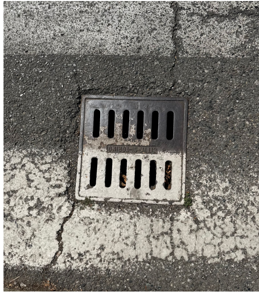
Figure 2.11: stormwater inlet identified along the mall boundary
