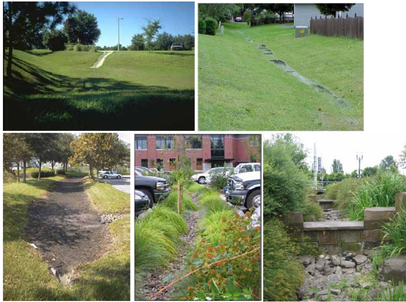
Figure 3.19: Examples of surface laminating structures consisting of open-air basins and channels [1]
