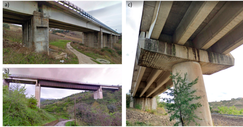
Figure 1.3: Different structural damages in (a) Typical PRC viaduct, (b) steel span of a viaduct and (c) circular piers with cap beam.
