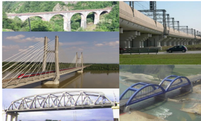
Figure 1.2: Bridges and viaducts maintained by RFI: several typologies made of masonry, r/c, p/c and steel
