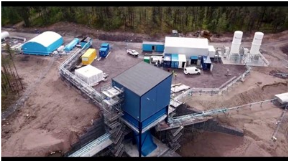
Figure 3.2: Test bench of company ISAR Aerospace — Credits: ISAR Aerospace
