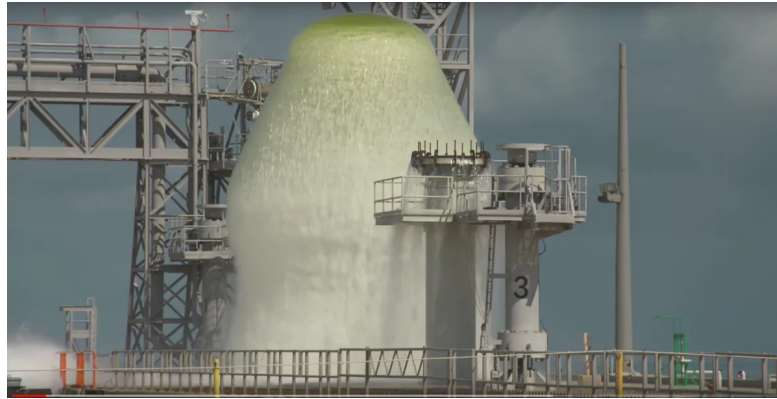
Figure 2.13: water deluge system on a launchpad (credits: NASA)
