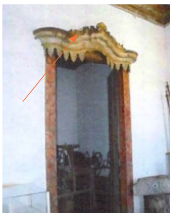
Decay: Soiling Possible Causes: Airflow patterns carrying dust and pollutants toward the top of the door; Poor indoor air quality or ventilation; Smoke from candles, cooking, or heaters; Condensation attracting dust in humid areas; Previous water infiltration leaving dirty marks; Improper or infrequent cleaning in hard-to-reach areas Location: Safena
