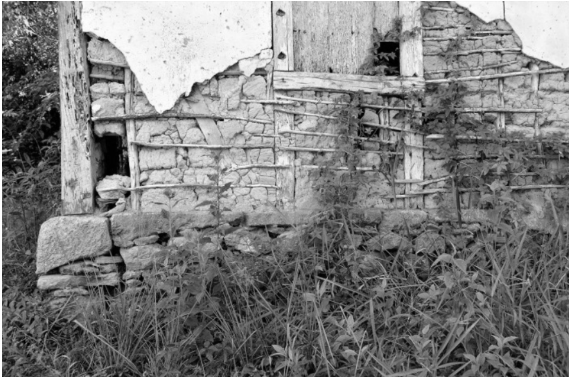
Figure 44 – External wattle and daub wall on stone foundation, Cachoeira do Brumado District, Mariana, MG, 2014. [Source: Image sourced from the website Vitruvius.]
