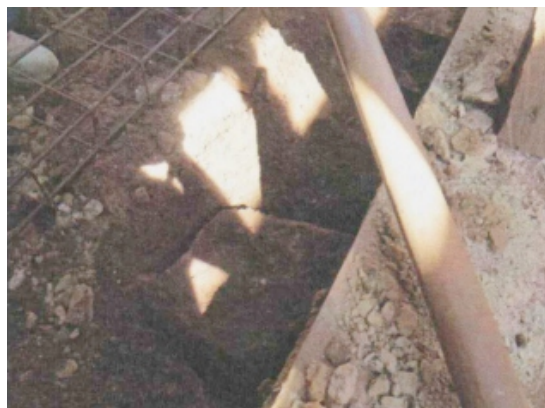
Repair and adding the stone foundation (type Ensilharia )
