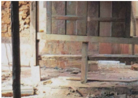
Wood replaced through the anchoring of the window.
