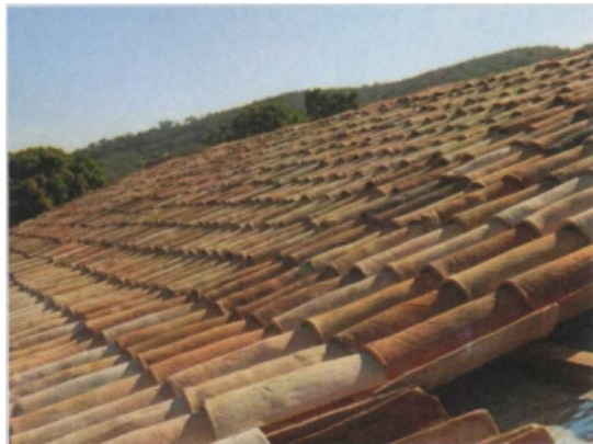
SC.EH. - Annex roof: simulating colonial tiles
