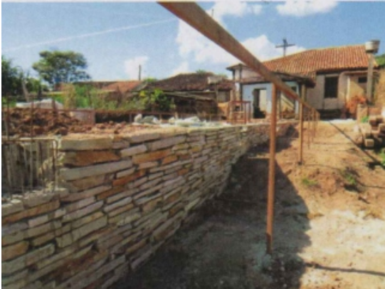
SC.EH. - Construction of the annex foundation in stone (Cangicado)
