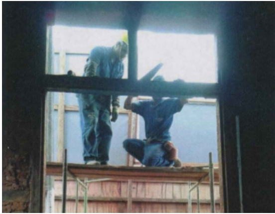
Removing the compromised elements
