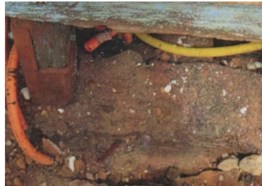
Foundations that had been replaced
