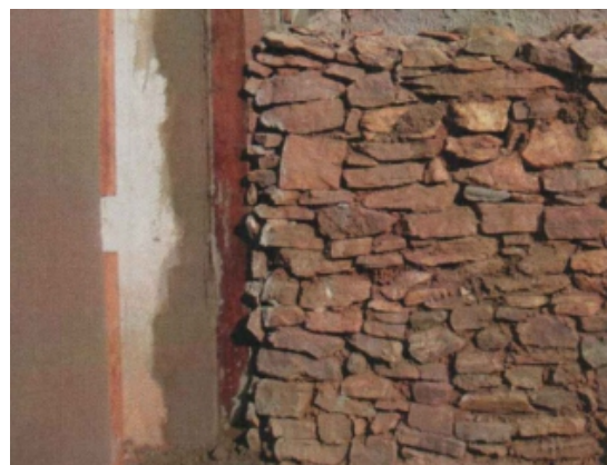
Adding the stone foundation (type Cangicado )
