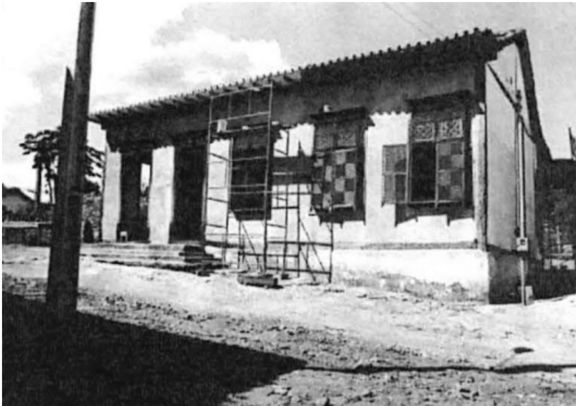
Figure 101 – Setecentista House during the restoration work in 1978. [Source: IPHAN-GO Collection.]
