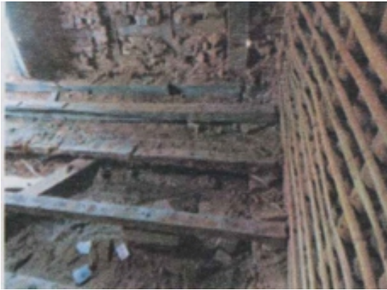
Careful removal of floor components (type Barrote)
