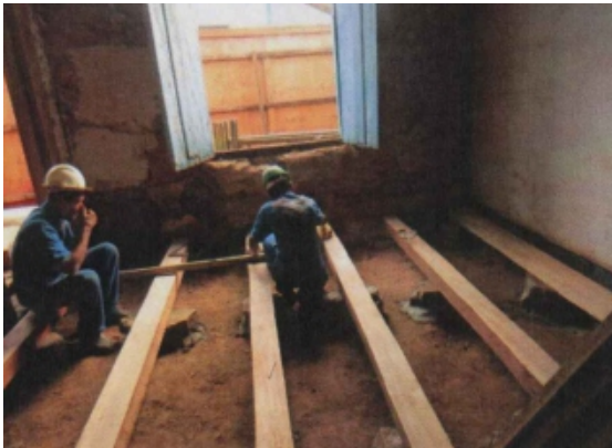
The complete replacement
