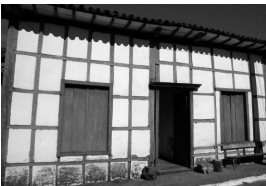
Figure 104 – Enxaimel House. [Source: GALVÃO, Marco Antônio. Pilar de Goiás, from the 18th to the 21st century. Vitruvius, year 2, no. 020.05, Oct. 2002.]
