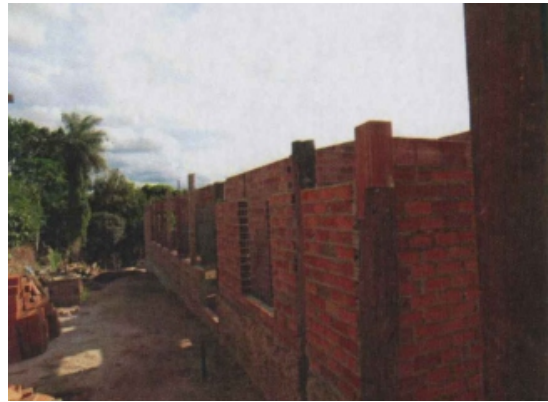
SC.EH. - Walls made of hollow bricks and cement
