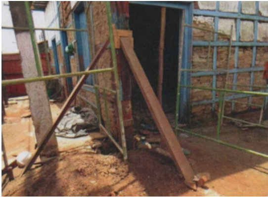
wood-borers and moisture were completely eliminated through the anchoring of the walls.
