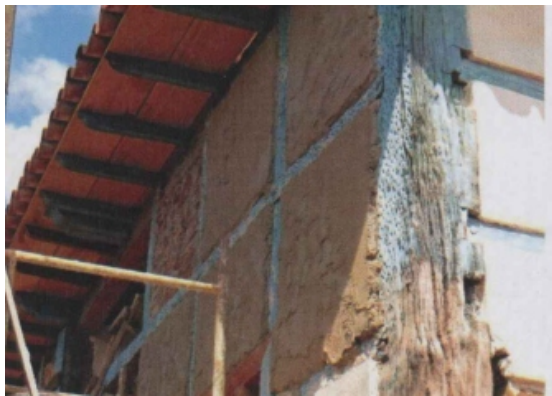
Applying the mortar on the walls
