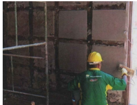
Application of lime paint
