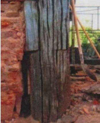
Decay: Wood-cracks Possible Causes: Loss of moisture causing contraction; Rapid or uneven drying; Internal stresses in the wood grain; Natural wood defects; Expansion and contraction cycles; Use of green wood; Mechanical stress or overloading; Aging and long-term weathering Location: Pillar
