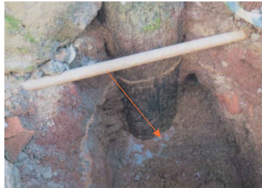
A survey was conducted on the house's foundations
