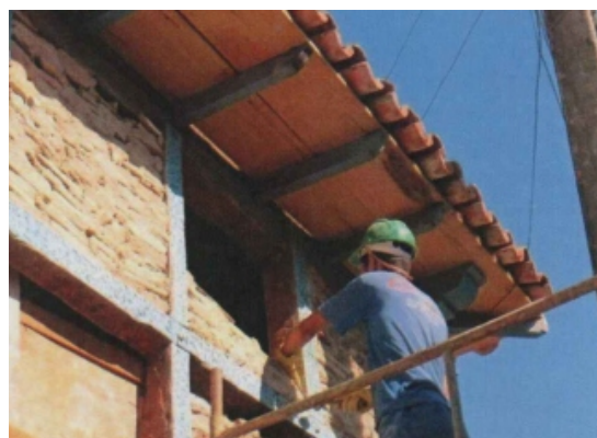
Total or partial reconstruction of the panels in the stone walls
