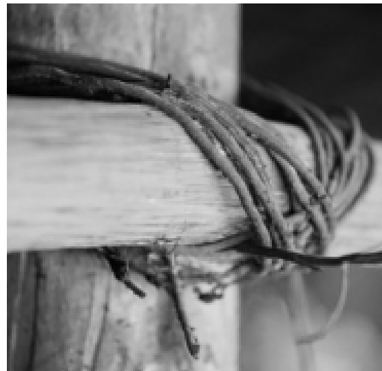
Figure 95 – Use of Titica Vine in Construction. [Source: Photograph by Marcos Amend, dated March 2019.]
