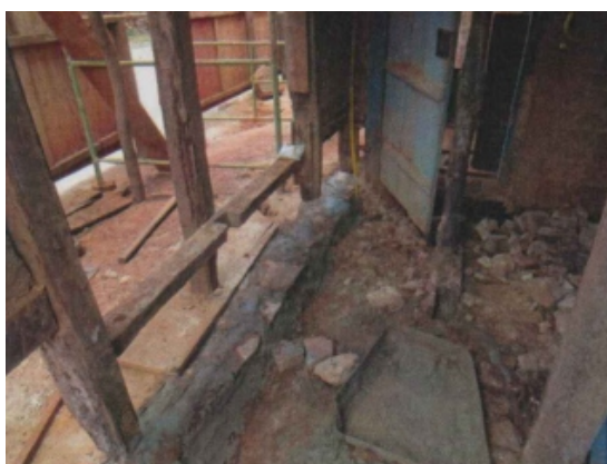
Repair the cement foundation (made in 1995)
