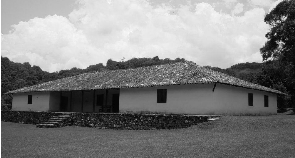
Figure 10 – Bandeirista House at Sítio Santo Antônio, São Roque, São Paulo, Brazil. [Source: Photograph taken on November 20, 2012, by José Augusto Bianchini.]
