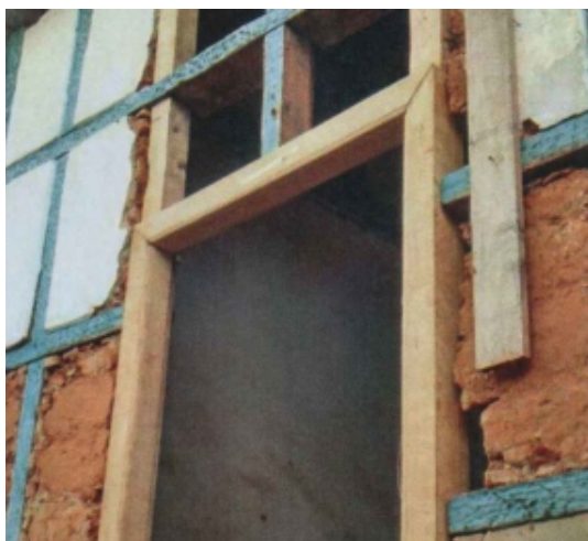
Adding the new wood elements
