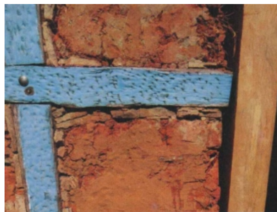
Controlled removal of damaged plaster for inspection and masonry repair
