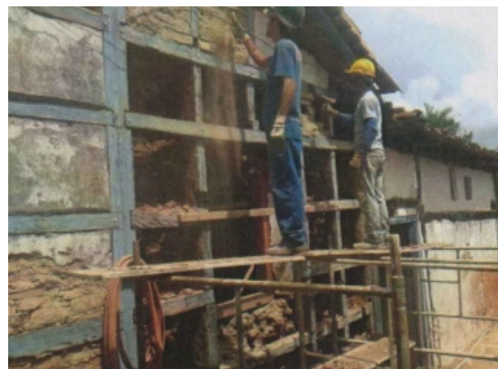
Controlled removal of damaged plaster for inspection and masonry repair
