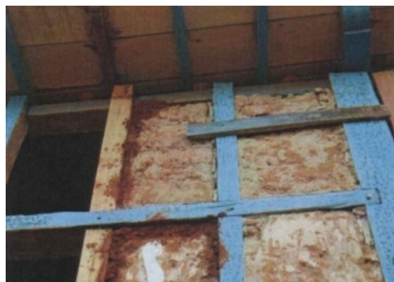
Clay filling in the adobe walls
