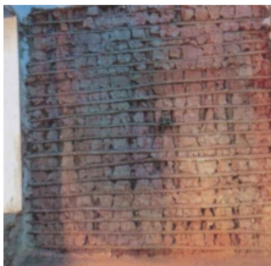
Controlled removal of damaged plaster for inspection and masonry repair
