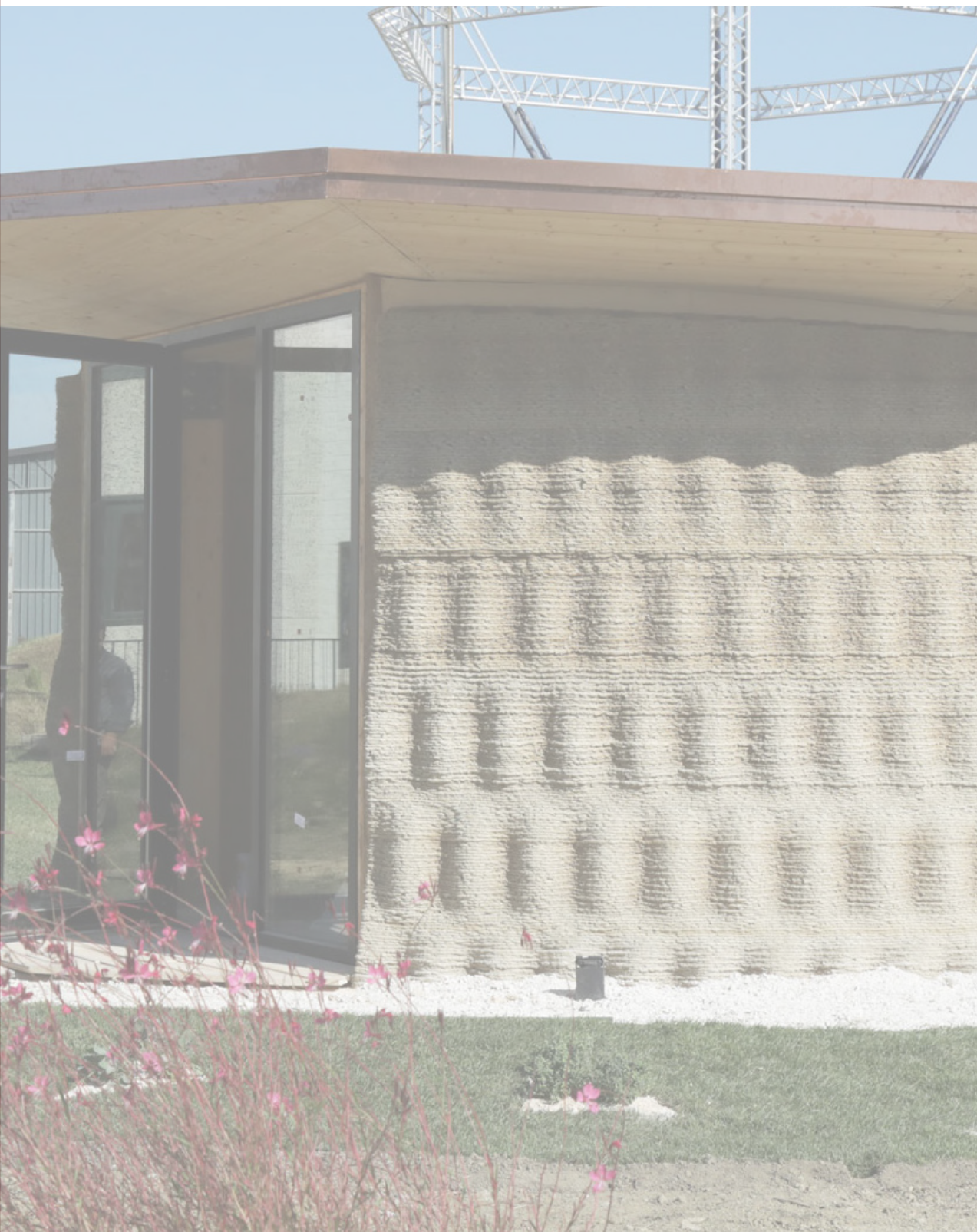
Fig. 124 Fotografia del modulo sperimentale stampato: GAIA https://www.3dwasp.com/wp-content/uploads/2018/09/3D-printed-house-Gaia-WASP-Italy-photo1_WEB.jpg
