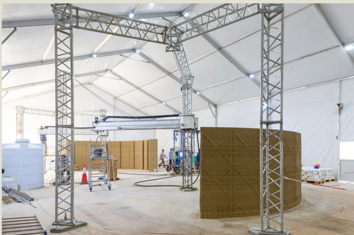
Fig 39. Crane Wasp in opera per la realizzazione del Dior concept store https://www.3dwasp.com/stampante-3d-per-case-crane-wasp/
