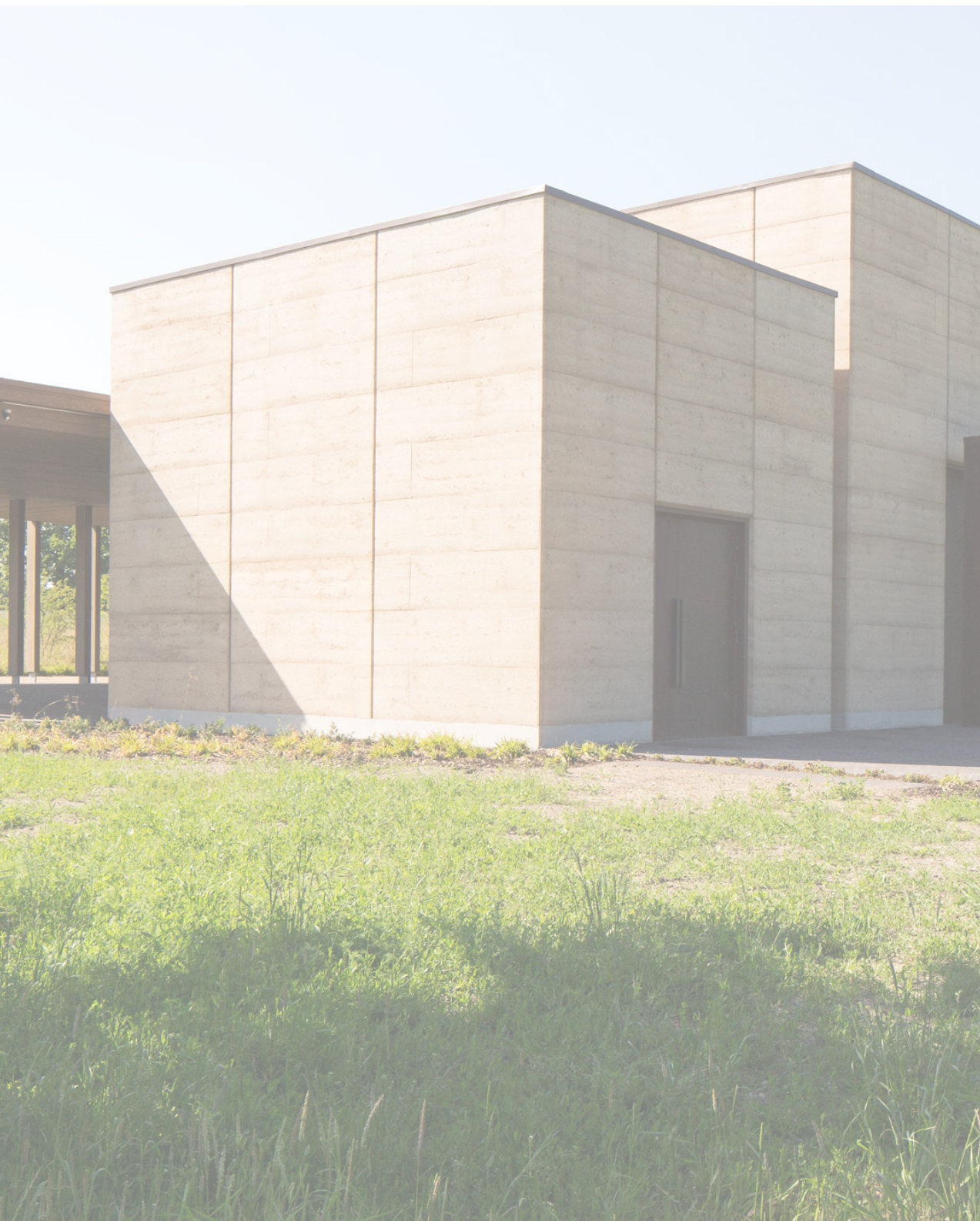
Fig 86. Sala preghiera cimitero Bushey. Fotografia di Lewis Kahn tratta da: https://www.dezeen.com/2017/11/22/waugh-thistleton-bushey-cemetery-rammed-earth-colonnade-extension-cemetery-hertfordshire-uk/#/
