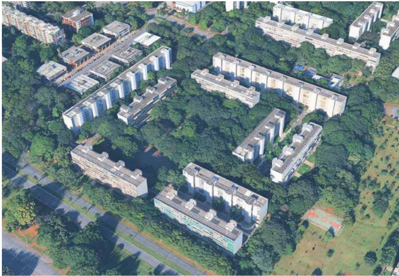
Figure 73: Perspective view of Superquadra 107 Norte, showing the difference in height of the buildings. Source: Google Earth, 2025
