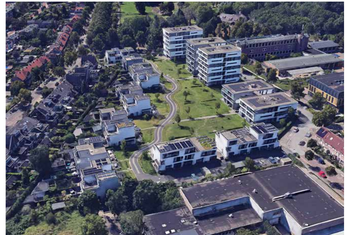
Figure 80: Aerial view of Frijhof-Housing, Netherlands . Source: Google Earth
