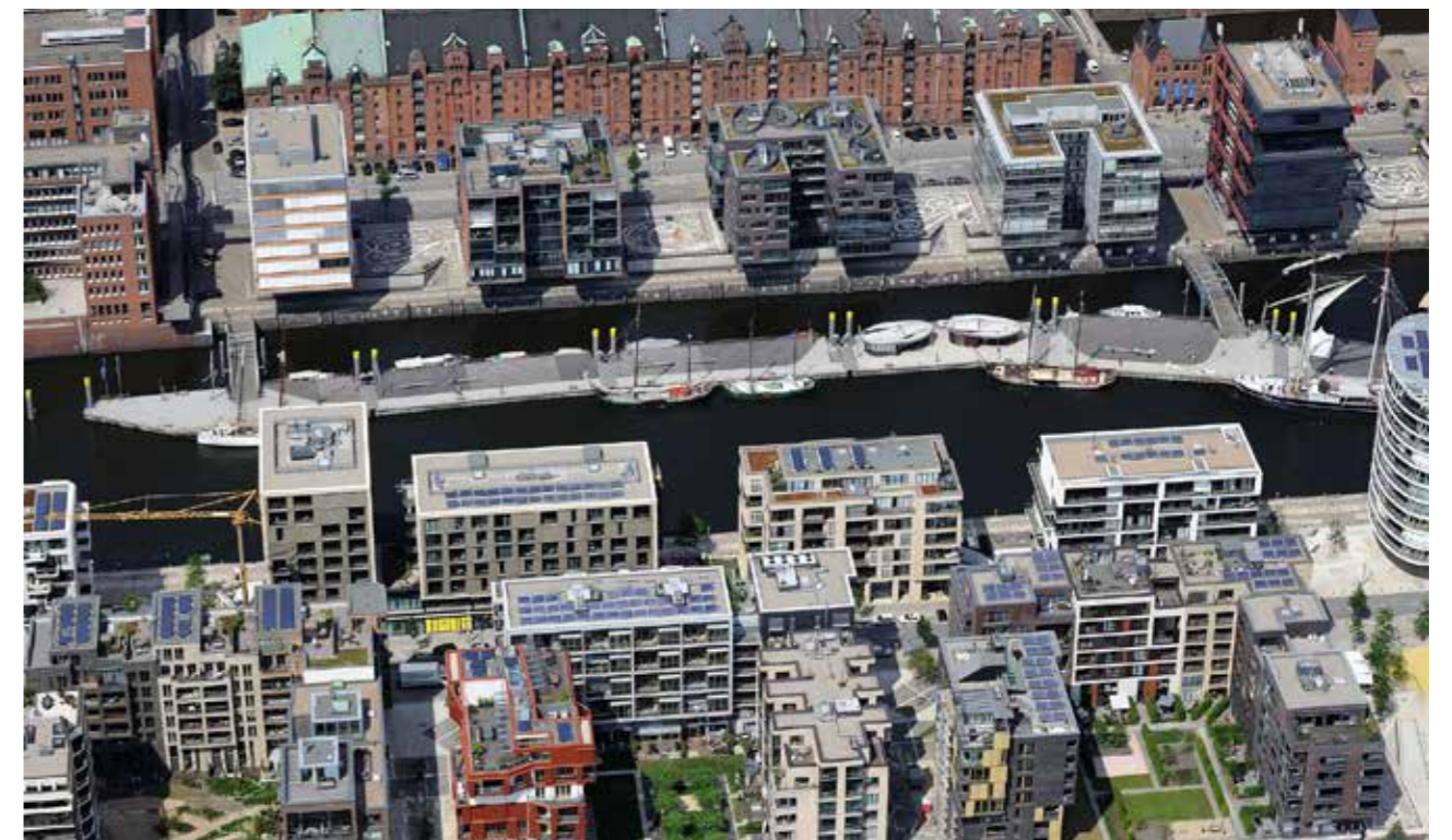
Figure 87: Aerial view of HafenCity, Germany. Source: KCAP
